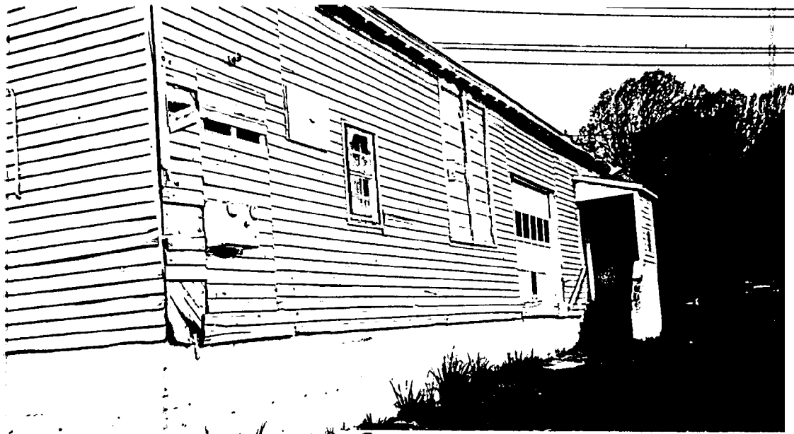
SMITHVILLE COLORED SCHOOL SOUTHEAST ELEVATION FROM ADJACENT PROPERTY
