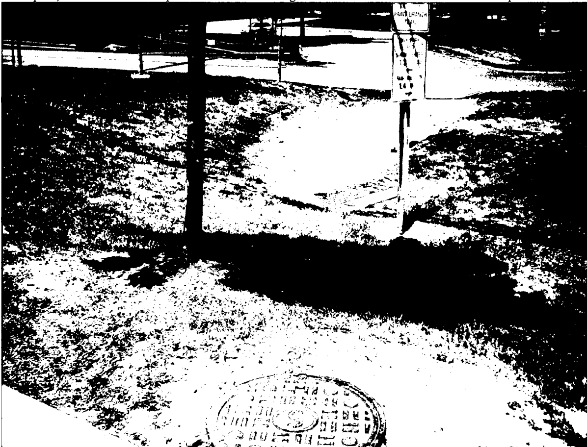
8-1-07 – looking NE, larger view of the stormdrain inlet area.
