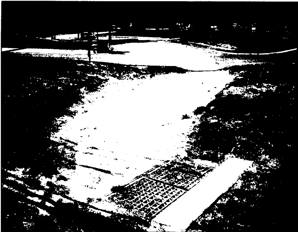
8-1-07 – looking NE, to existing inlet and asphalt swale to be changed out to a flat, grass swale. The asphalt is from the old driveway to the park, and all the visible asphalt and associated subgrade shown above will be removed and replaced with compost and soil.
