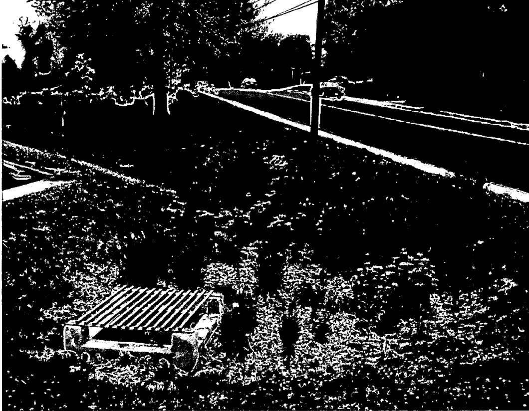
Example of vegetated swale at the Dennis Ave. Health Center (note - Valley Mill be more densely vegetated and outfalls will discharge into existing drainage).
