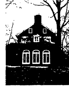
4 West Elevation of Hayes Manor
