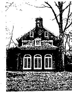
4 West Elevation of Hayes Manor
