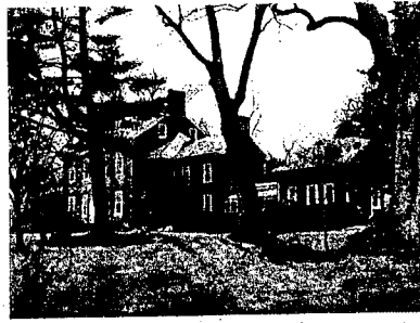
2 East Elevation of Hayes Manor
