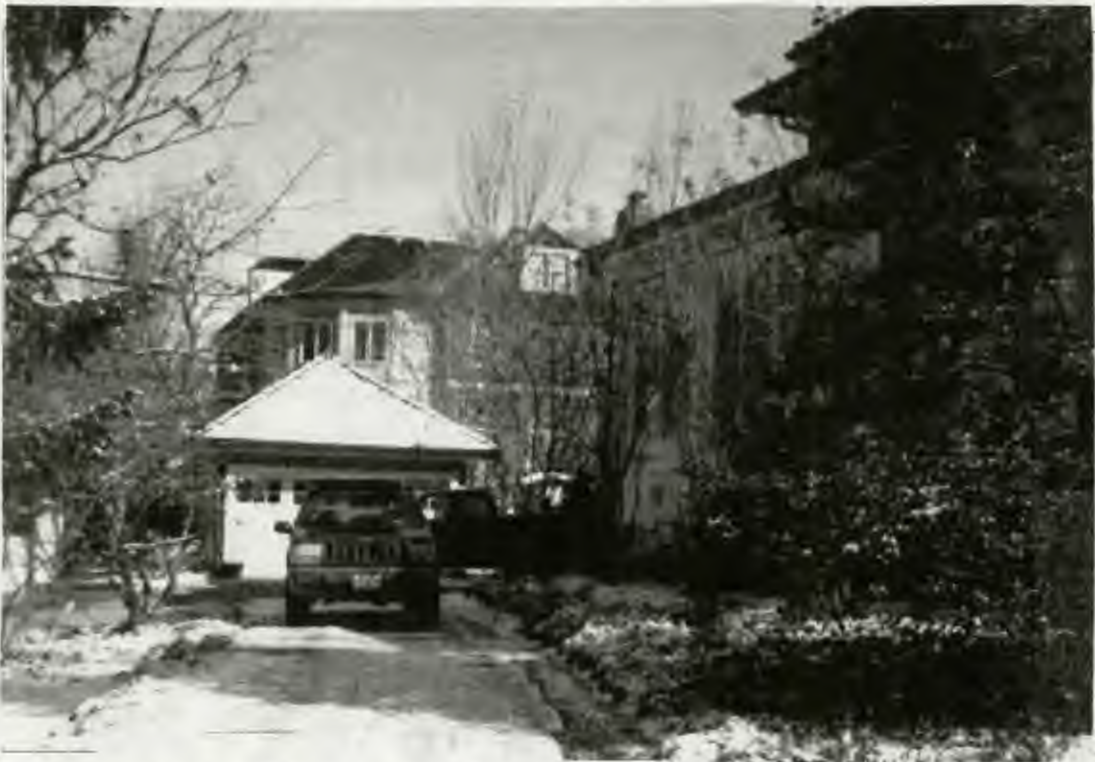
Detail: View Towards Garage and Rear Property Line
