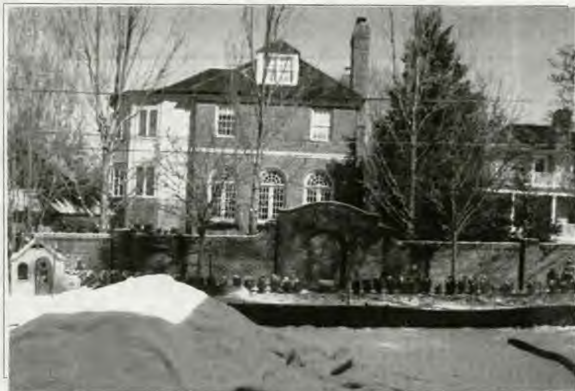
Detail: View Looking North, Towards rear property line.
