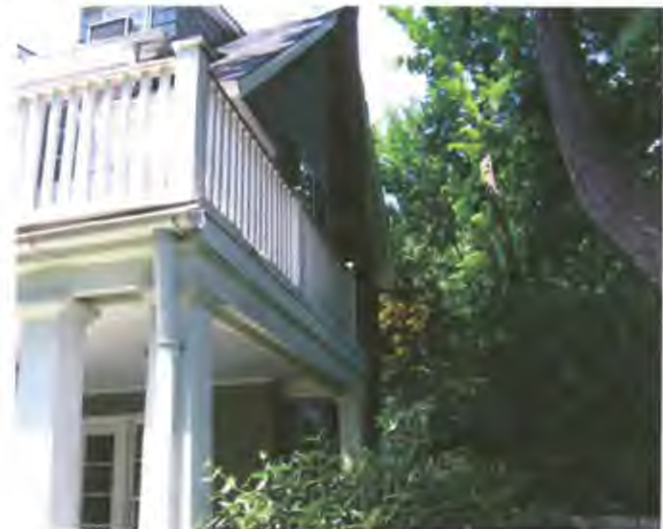
EAST FACADE FROM ADJOINING PROPERTY
