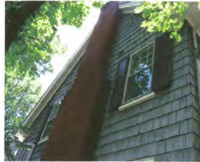
EAST FACADE FROM ADJOINING PROPERTY
