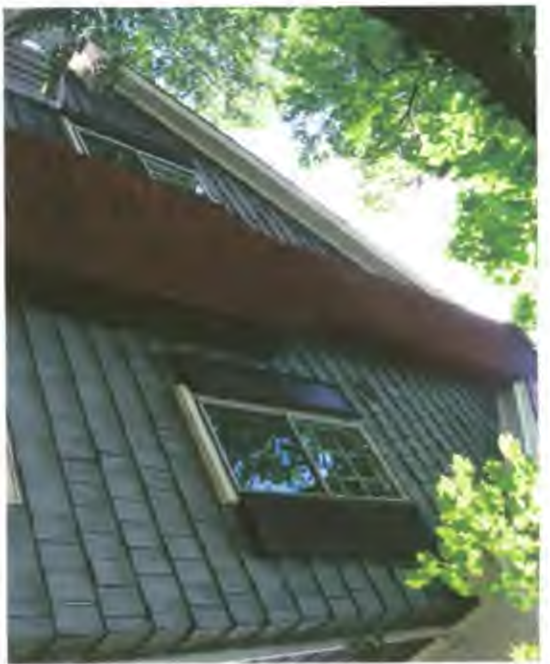
EAST FACADE FROM ADJOINING PROPERTY
