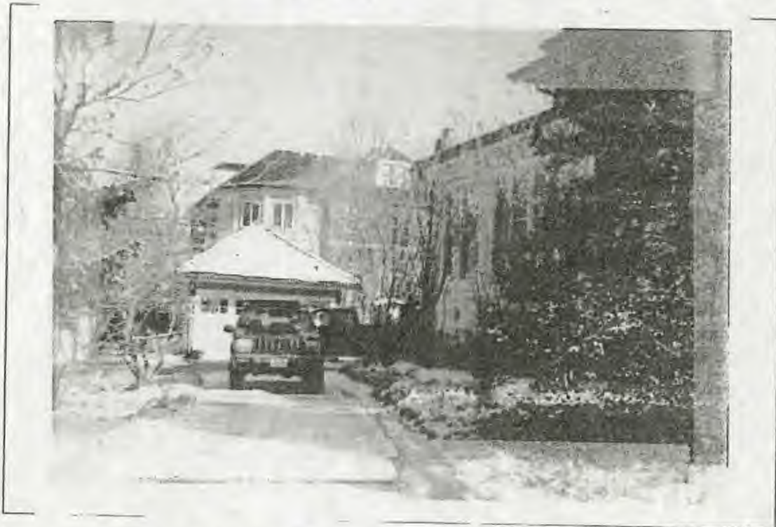
Detail: VIEW TOWARDS GARAGE AND REAR PROPERTY LINE
