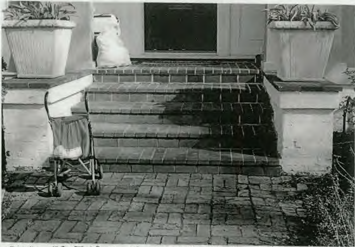
Detail: FRONT VIEW OF EXISTING STEPS and WALK
