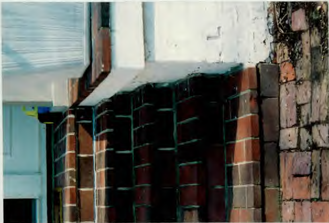
Detail: PARTIAL FRONT VIEW OF EXIST'G. STEPS
