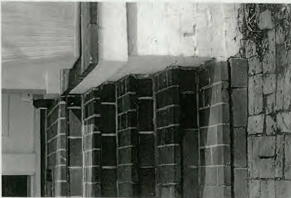
Detail: PARTIAL FRONT VIEW OF EXIST'G. STEPS
