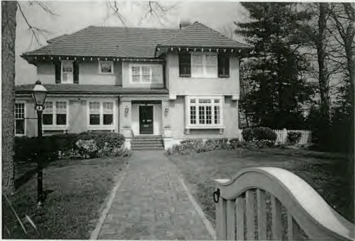
Detail: VIEW OF FRONT OF HOUSE FROM SIDEWALK
