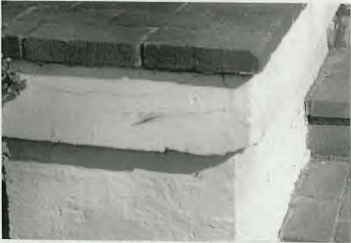
Detail: TOP OF EXISTING MASONRY PIER
