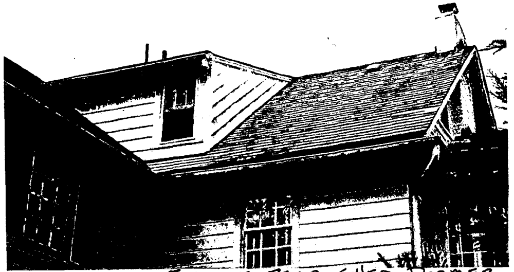
EXISTING REAR SHED DORMER
