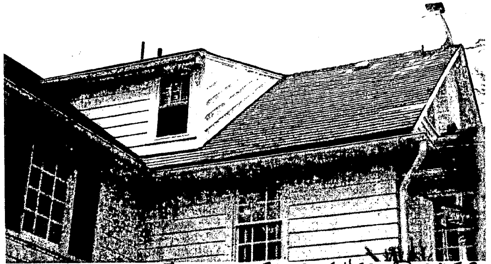
EXISTING REAR SHED DORMER
