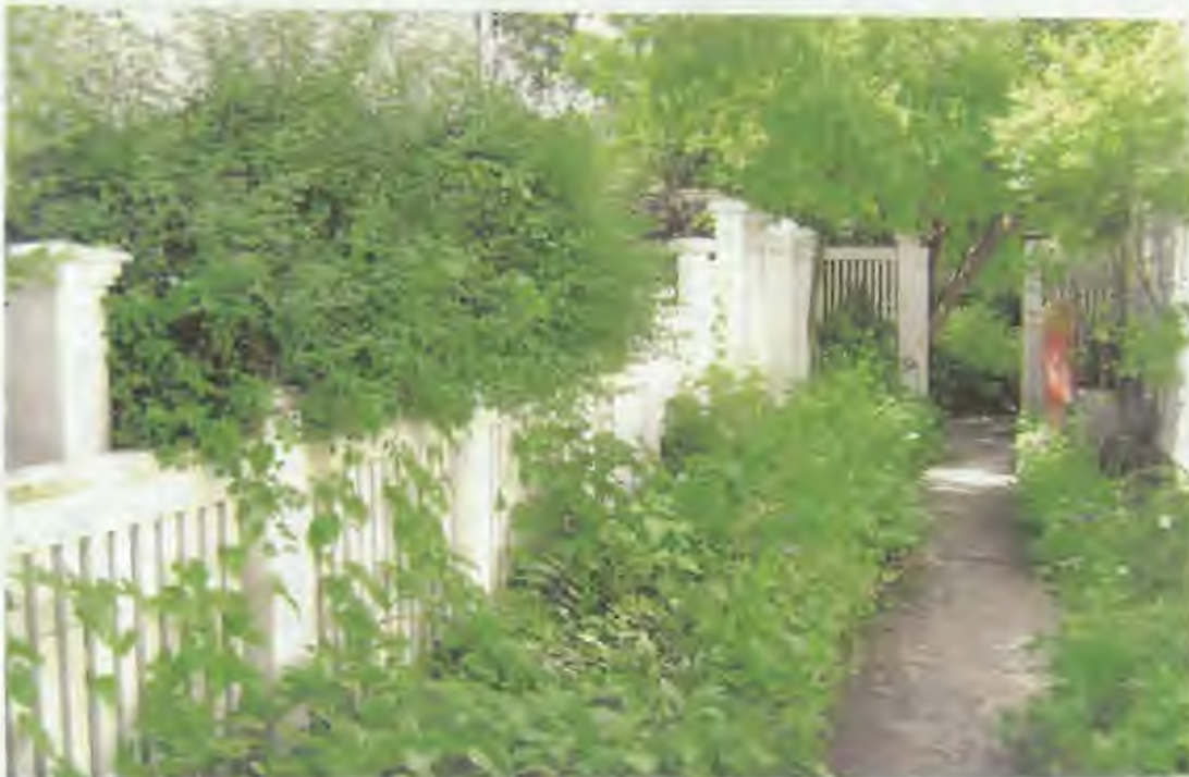
Detail: LEFT FRONT (EAST FENCE)
