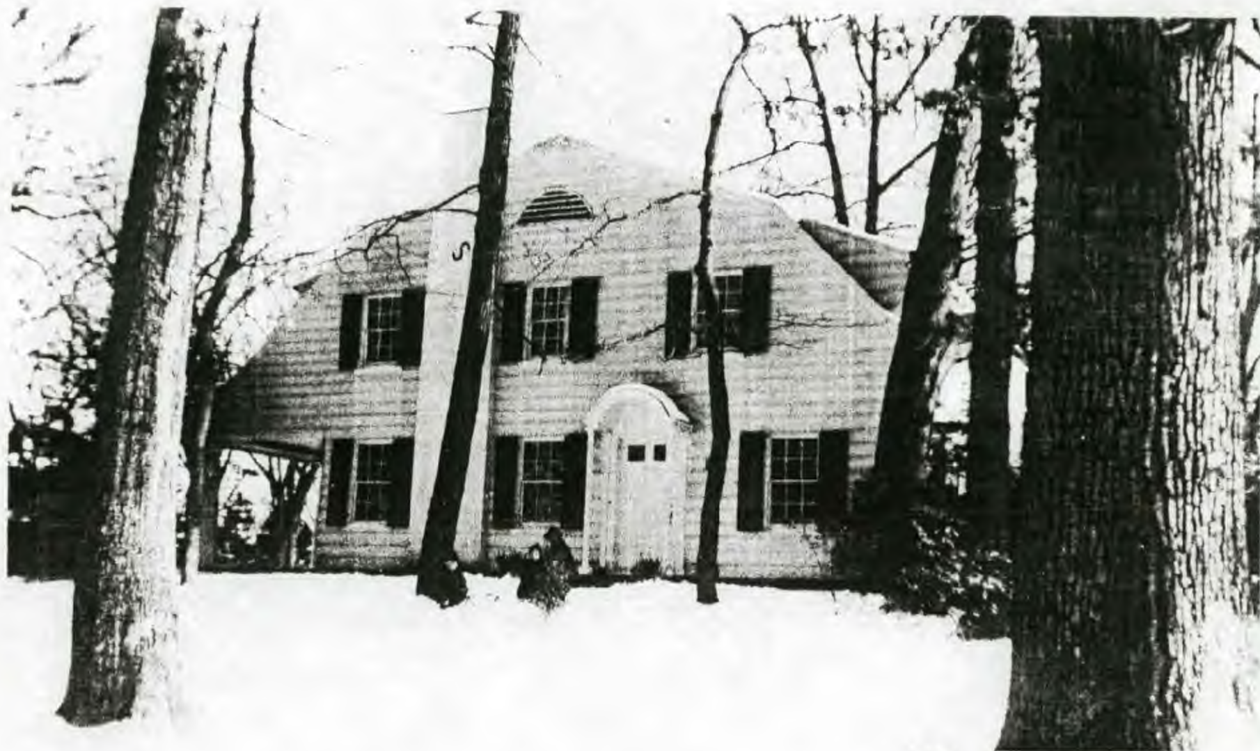
#18 8 Newlands Street Original West Façade Prior to 1990 Addition
