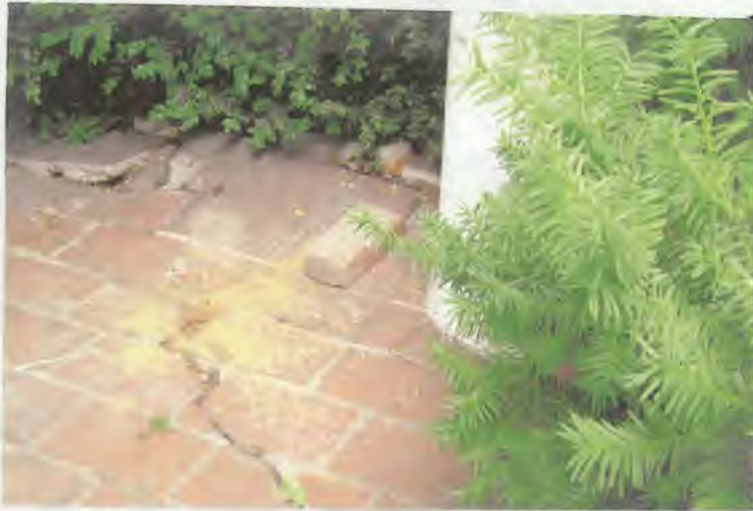
Detail: PORCH LEFT FRONT
