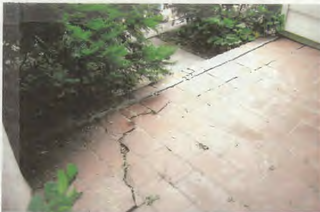
Detail: PORCH CENTER
