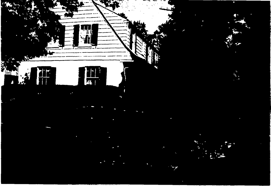
Detail: 13 OXFORD STREET, View FROM Public Street, camera facing North
