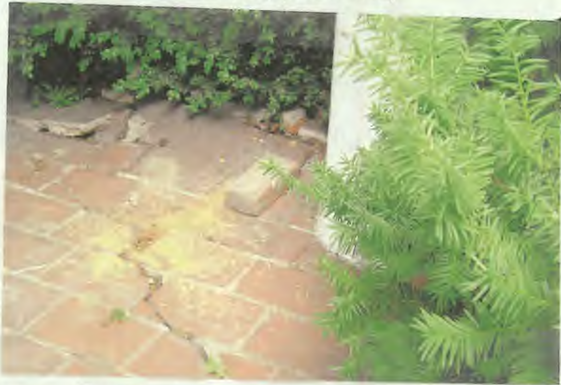
Detail: PORCH LEFT FRONT
