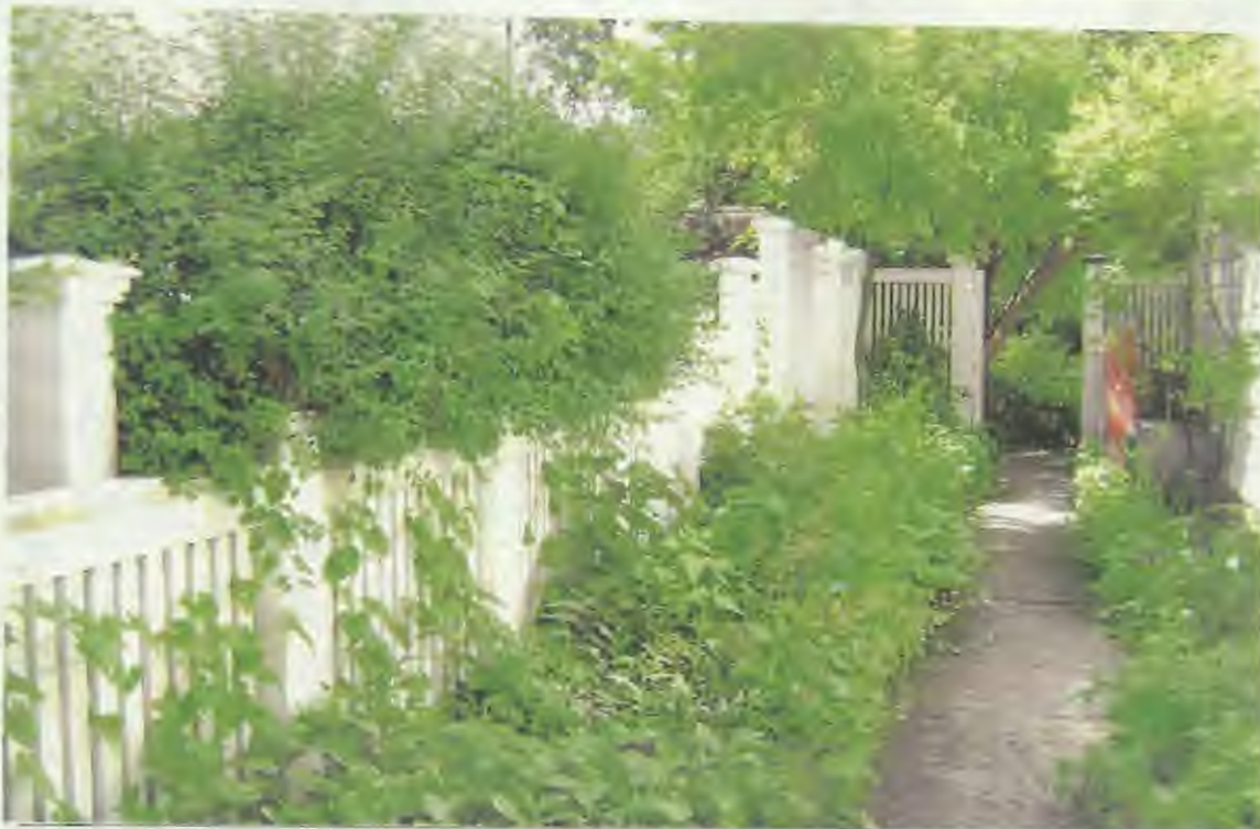
Detail: LEFT FRONT (EAST FENCE)
