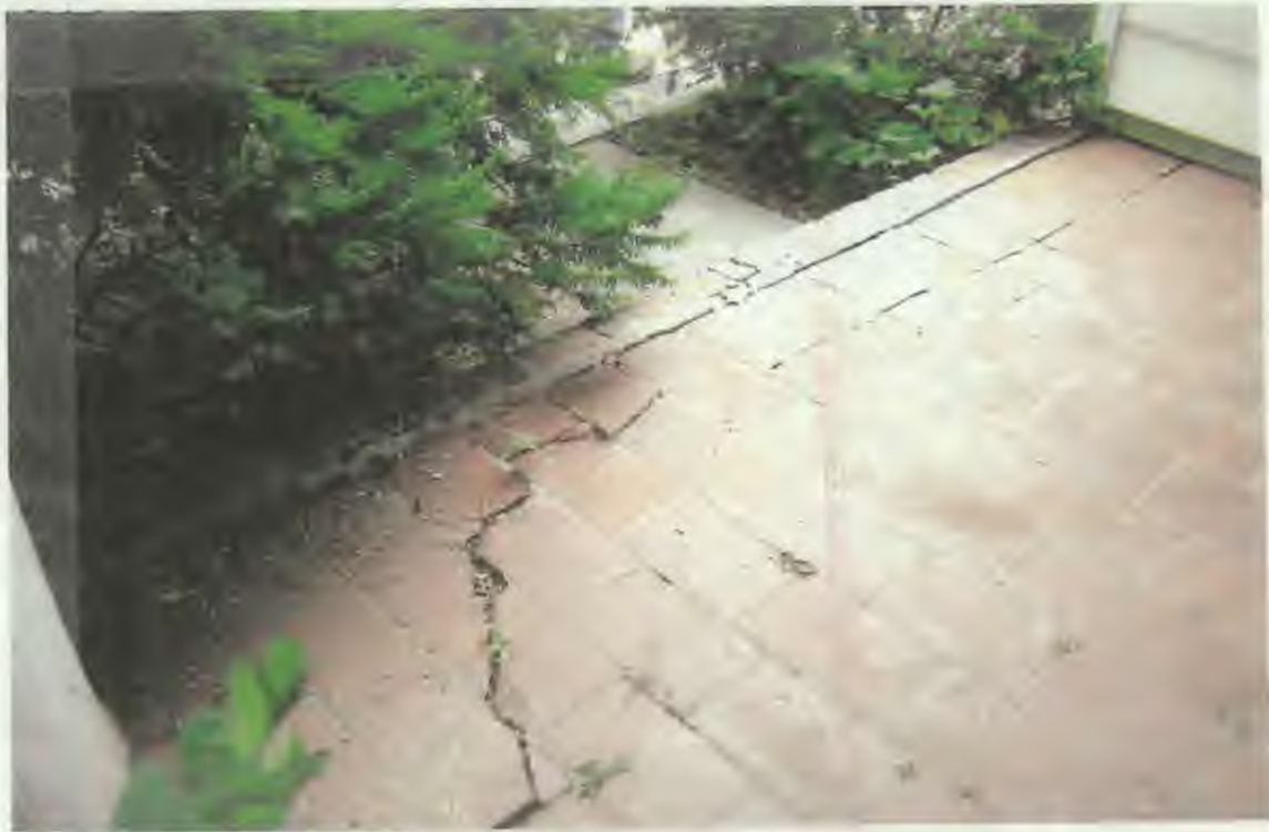
Detail: PORCH CENTER
