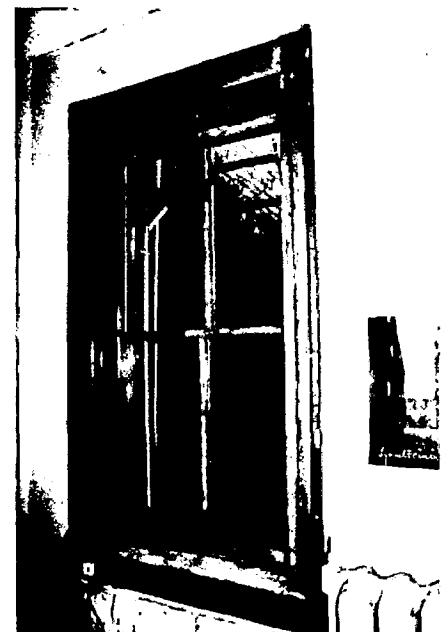
Figure 4f. Following the relatively simple repairs, the window is weathertight, like new in appearance, and serviceable for many years to come. Both the historic material and the detailing and craftsmanship of this original window have been preserved. Photo: John H. Myers
