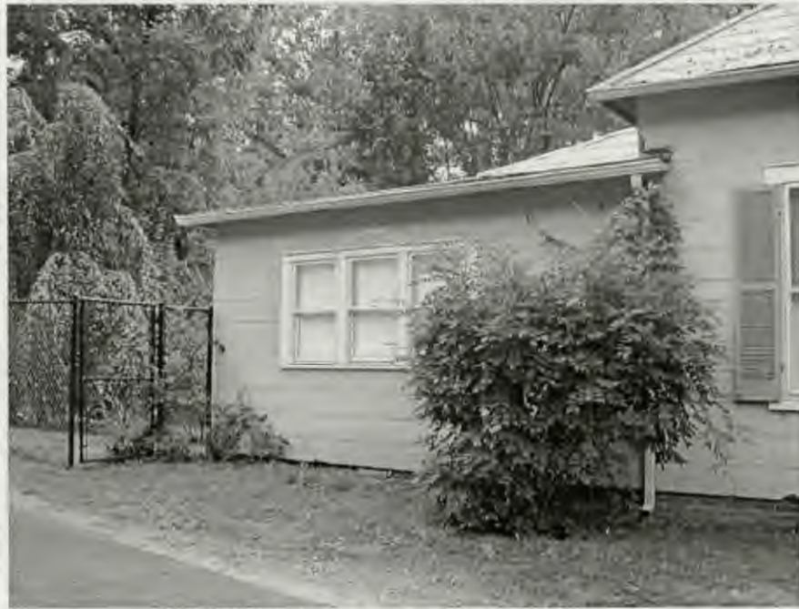
7108 Holly Ave., rear addition on south side
