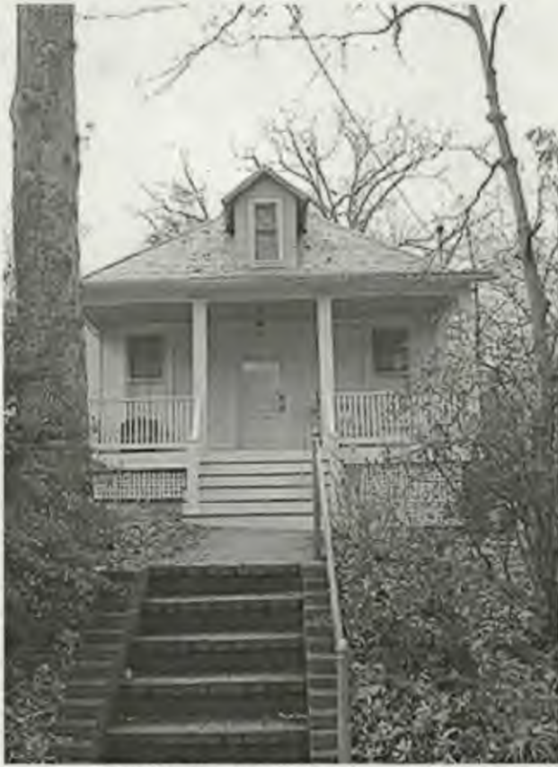
7108 Holly, front view from street
