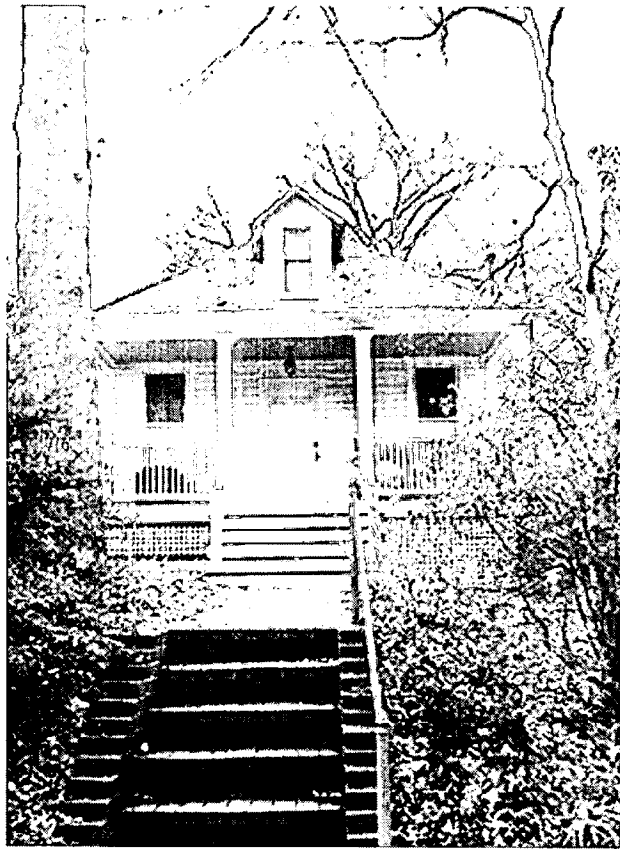
7108 Holly, front view from street
