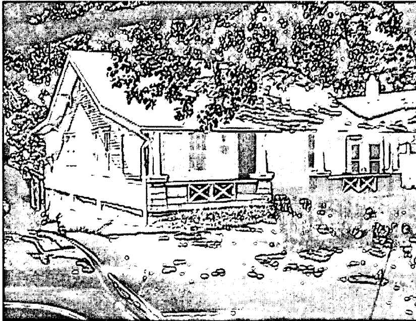
242 Park Ave. (front view)
