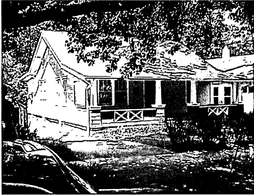
242 Park Ave. (front view)
