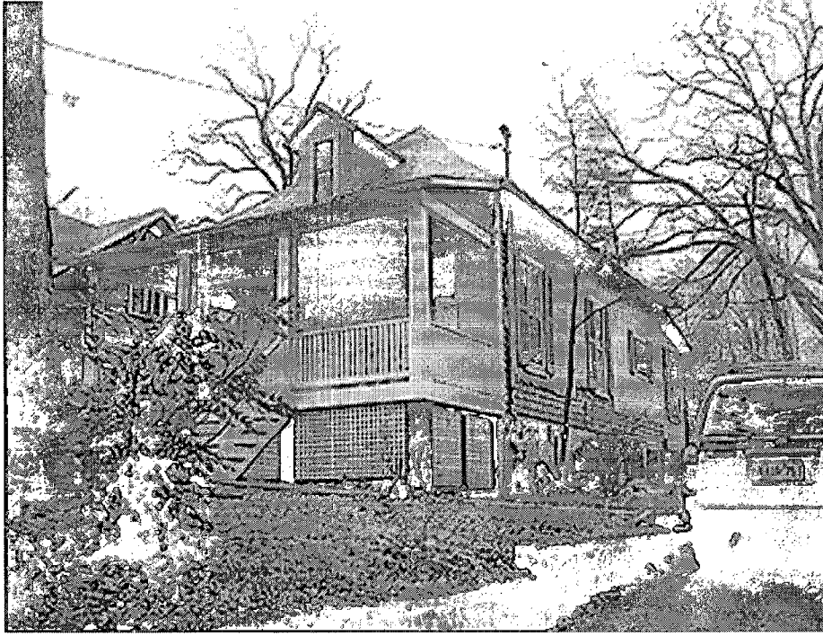
7108 Holly Ave., north side
