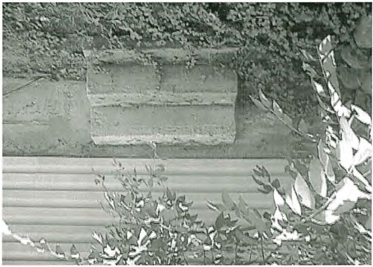
Side step for door in carriage house
