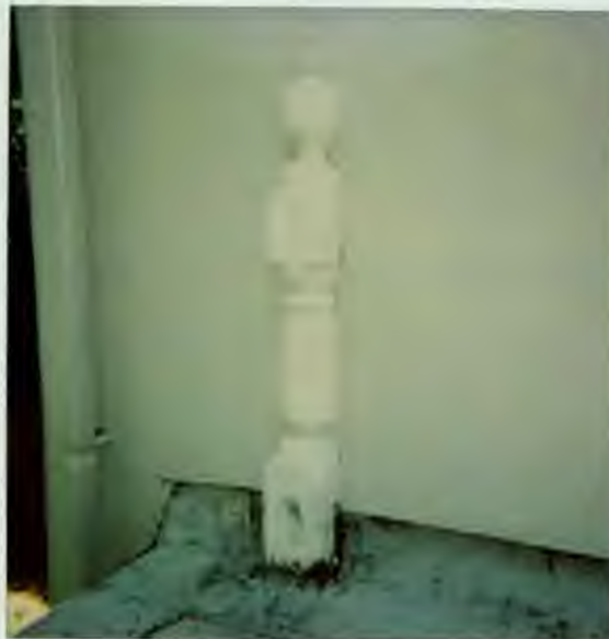
PARTAN RESIDENCE 25 HOLT PL NEWEL @ FRONT PORCH ROOF SIM. TO 1930'S PHOTO
