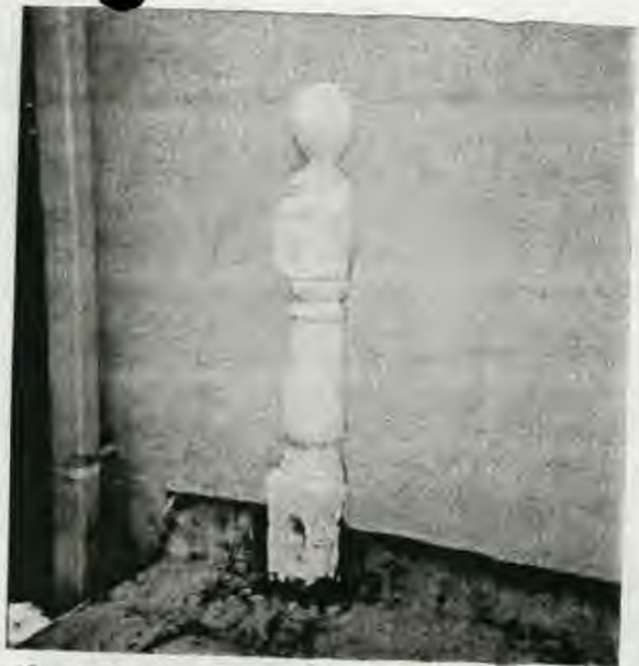
PARTAN RESIDENCE 25 HOLT PL NEWEL @ FRONT PORCH ROOF SIM. TO 1930'S PHOTO
