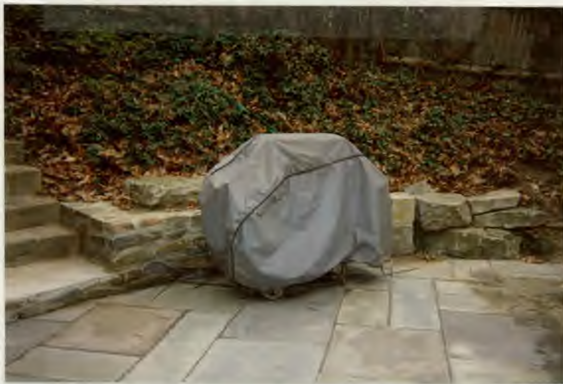
Stone wall, east of existing steps
