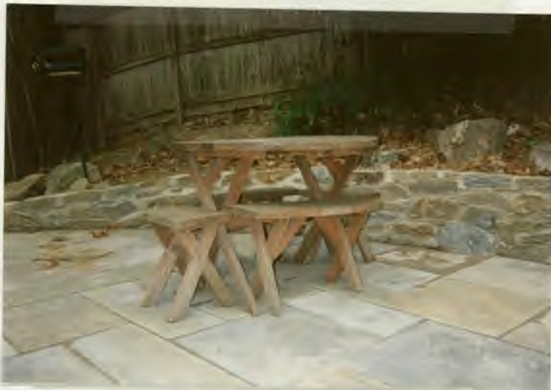
Stone wall, left of existing steps (west)
