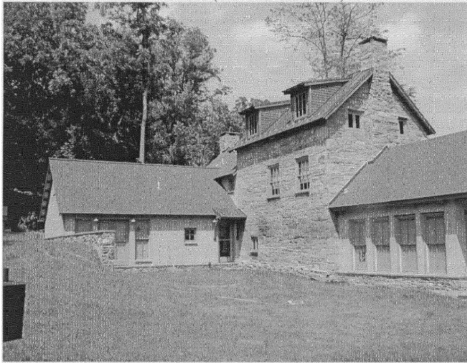
side view of house (addition site)
