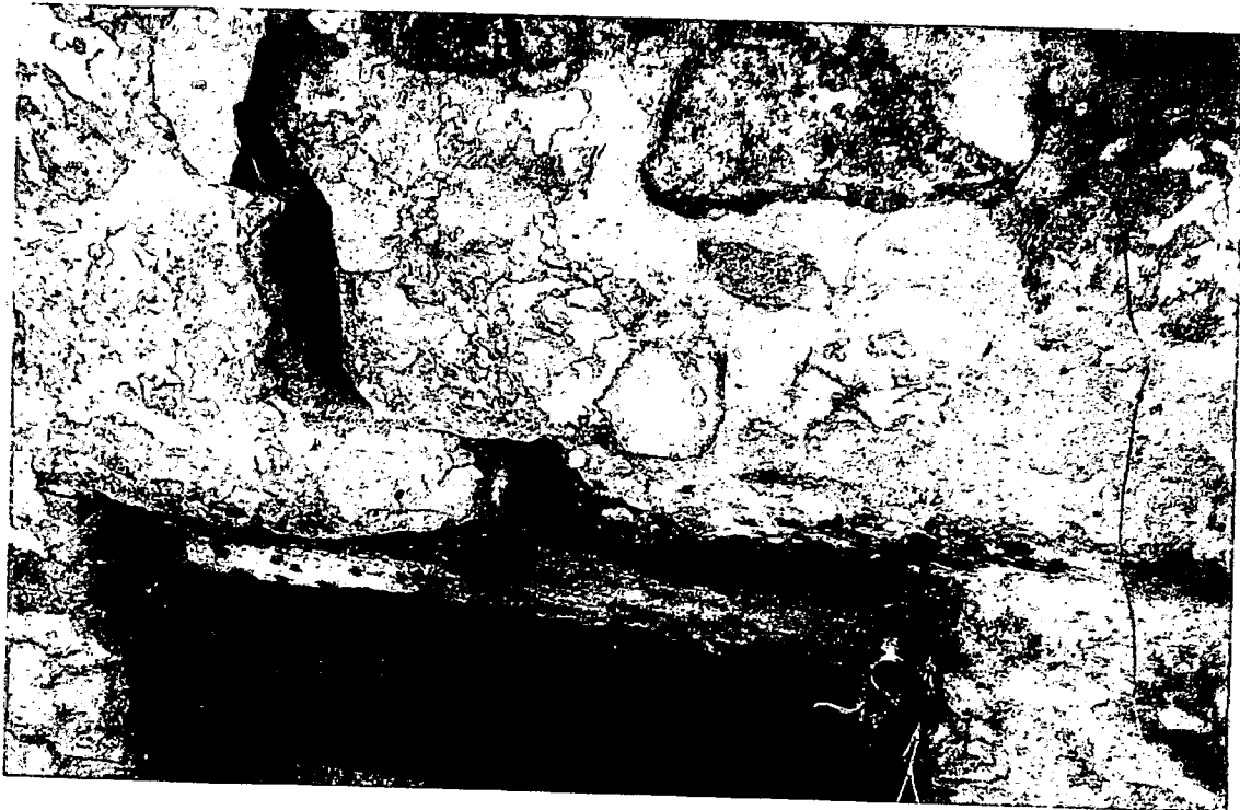
2. Three inch wide crack in east wall due to outward and southward movement.
