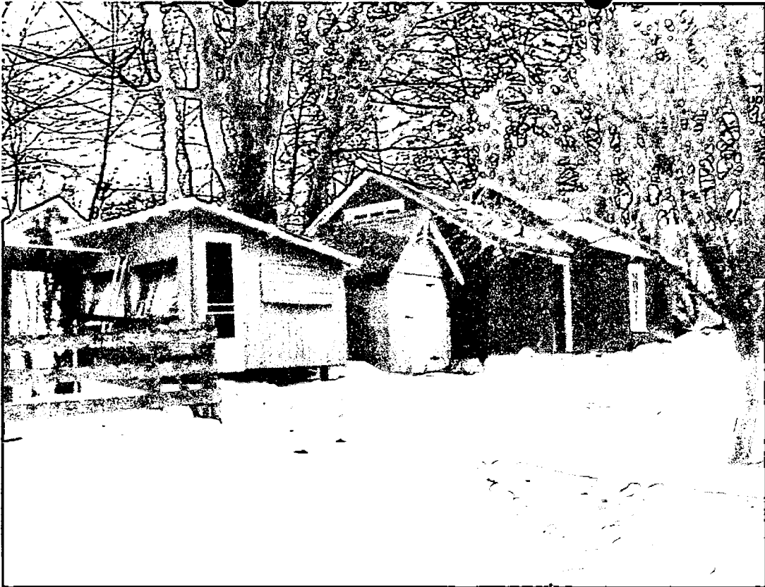
East Elevation - Including Other Outbuildings
