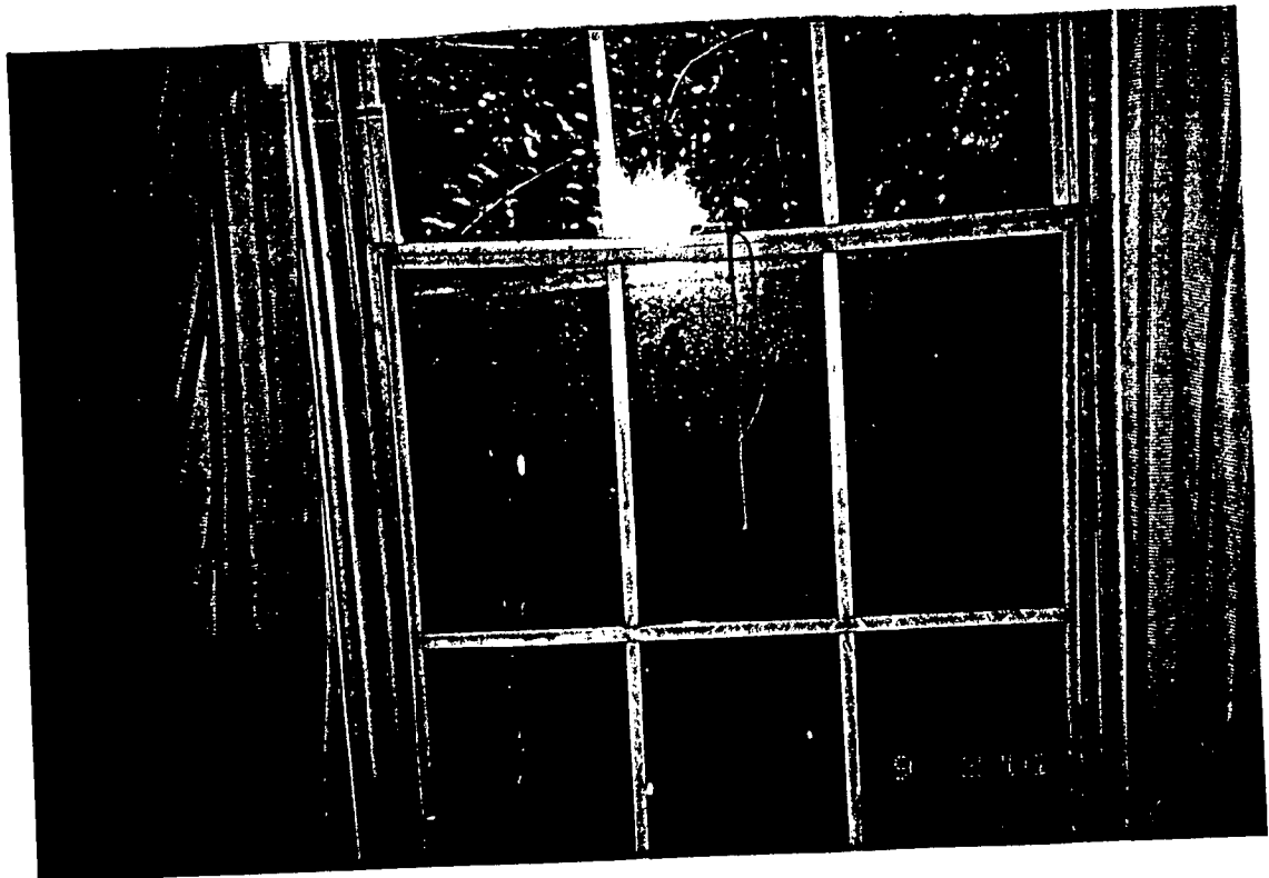
Distorted Window, wired together with coat hanger
