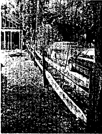
1.) existing bottom half of fence Between property 310 & 312.
