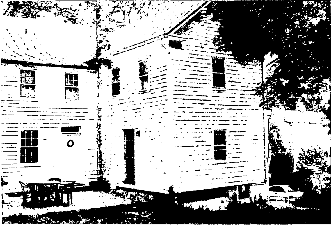
Detail: South west current view of L-wing
