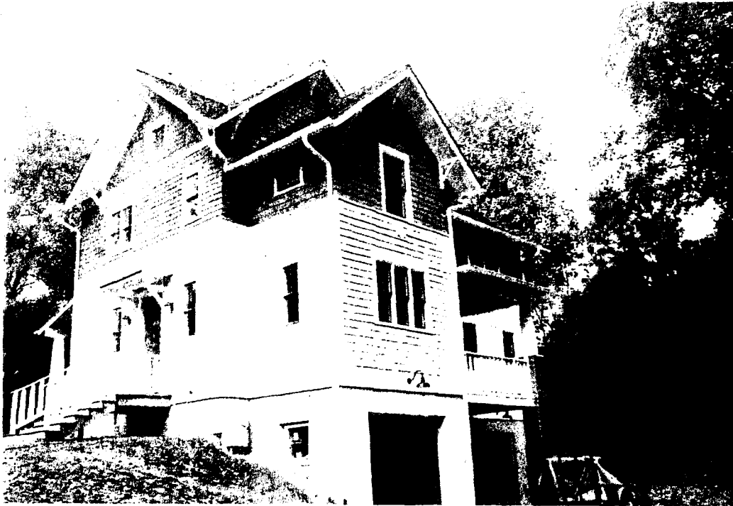
Detail: Example of triple and single double overhung splitpane, East of 201 Market Street
