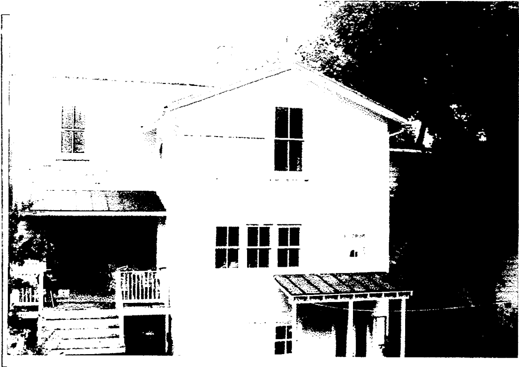
Detail: Example of triple awning windows, rear of 8 Market Street
