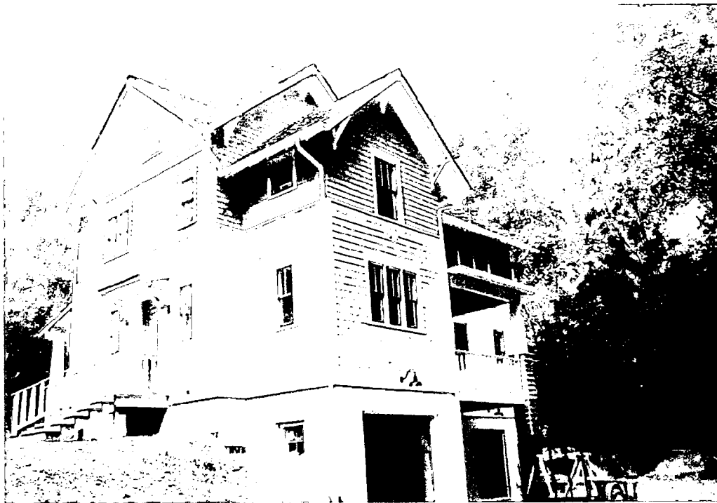
Detail: Example of triple and single double overhung split pane, East of 201 Market Street
