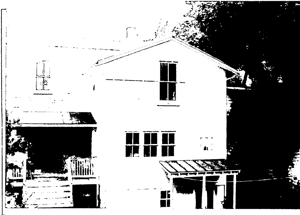
Detail: Example of triple overhung windows, rear of 8 Market Street
