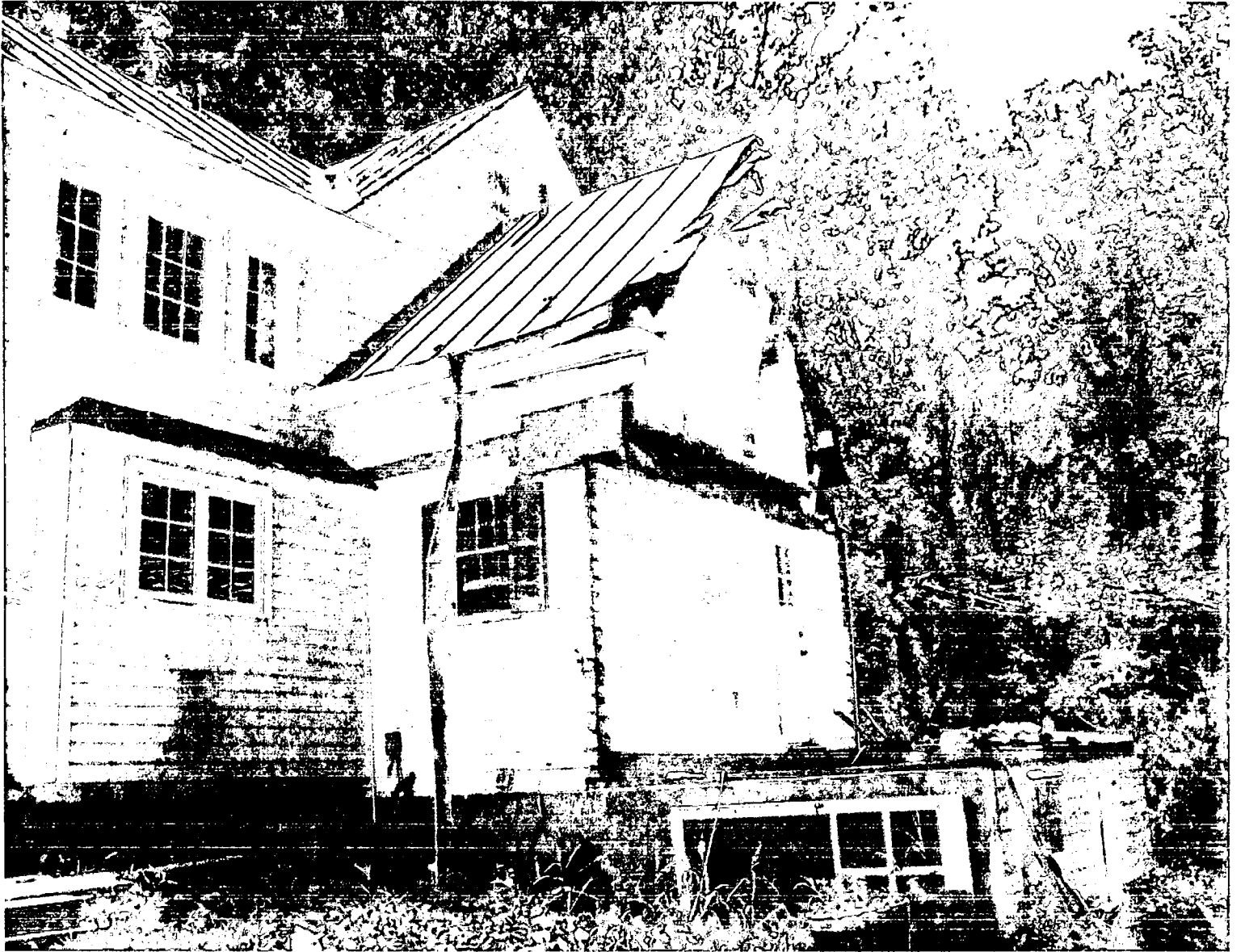
REAR COURT VIEW - CURRENT .
