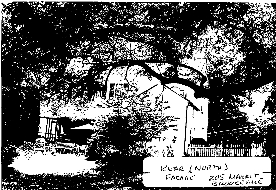
Detail: REAR (NORTH) FACADE SHOWING KITCHEN ELL
