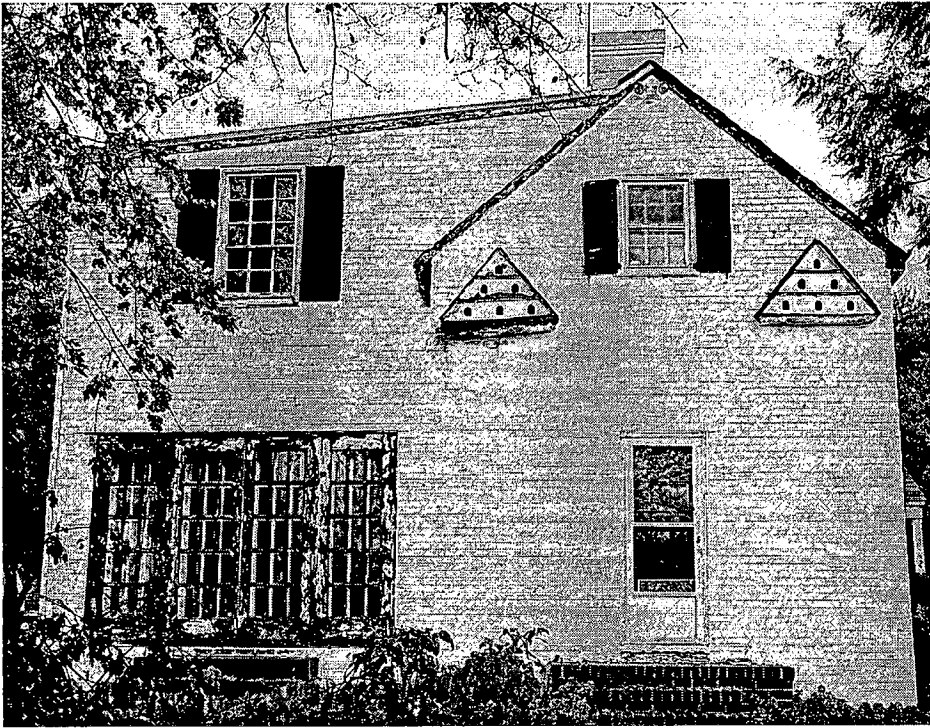
Building A South Elevation October 24, 2003 ca. 1939 brick addition
