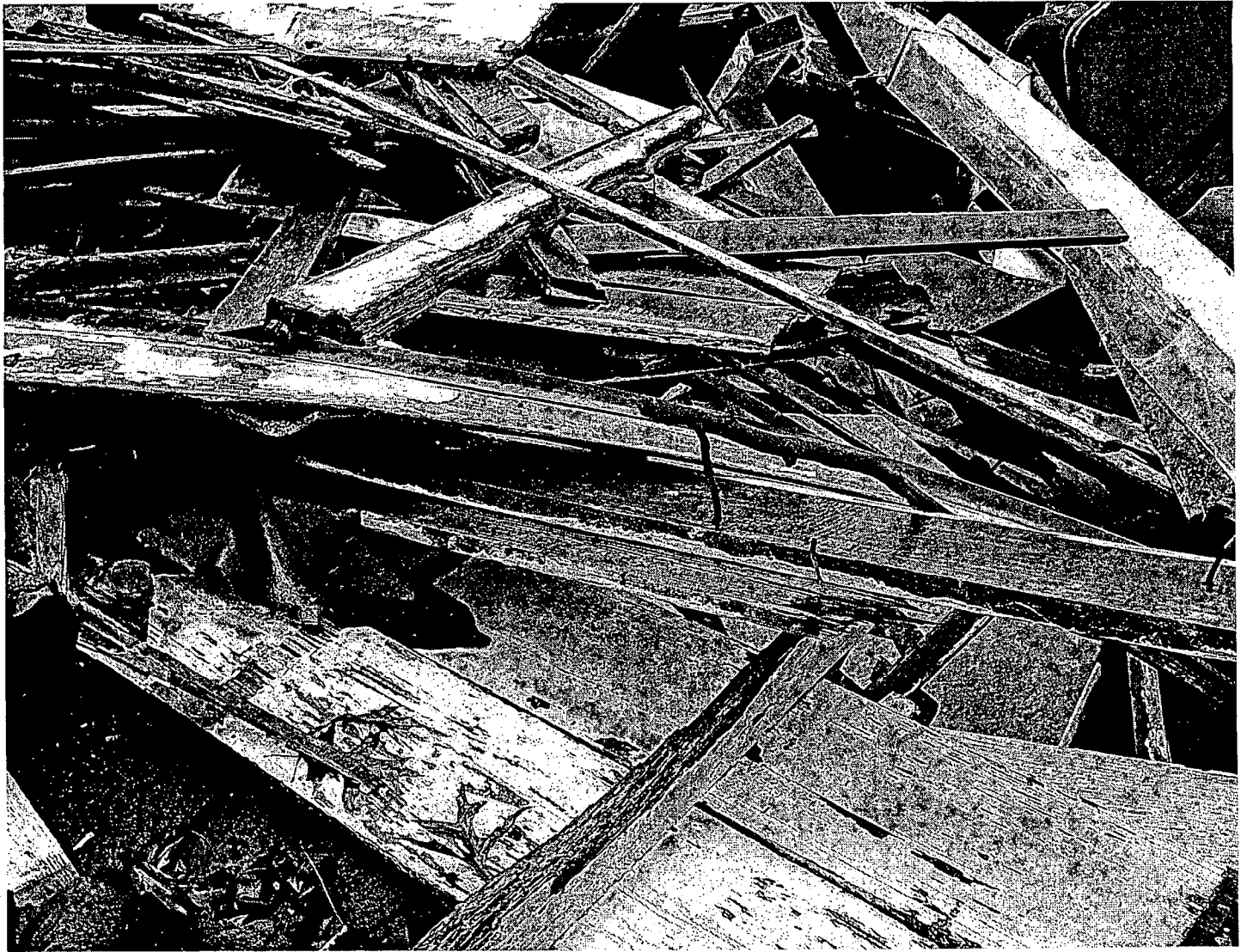
Building E Debris Pile Closeup Showing fencing and clapboard removed and stacked. October 24, 2003
