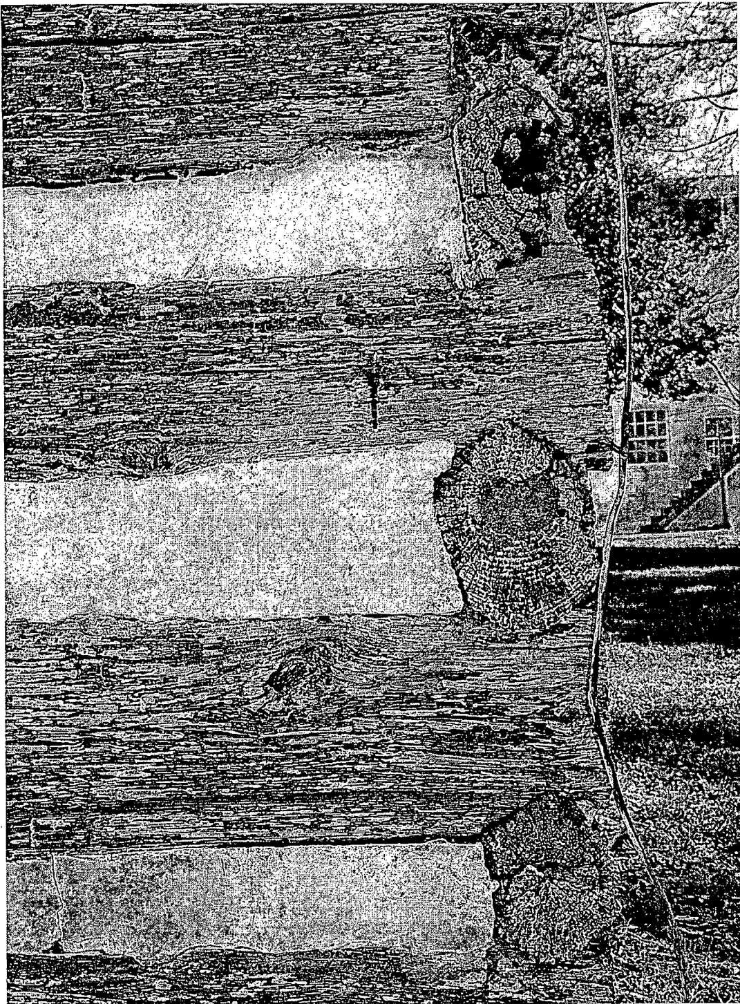
Building D V-notch logs Smokehouse Nov. 2003
