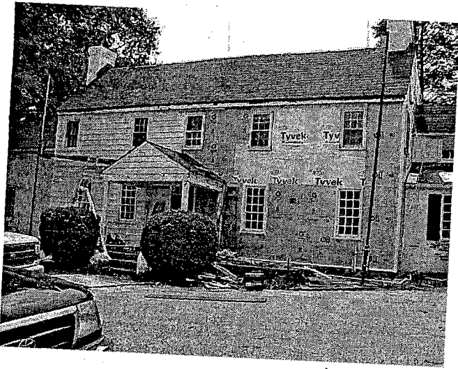
Building A Summer 2003
