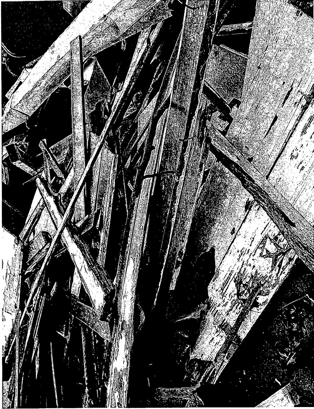
Building E Debris Pile Closeup Showing fencing and clapboard Removed and stacked, October 24, 2003
