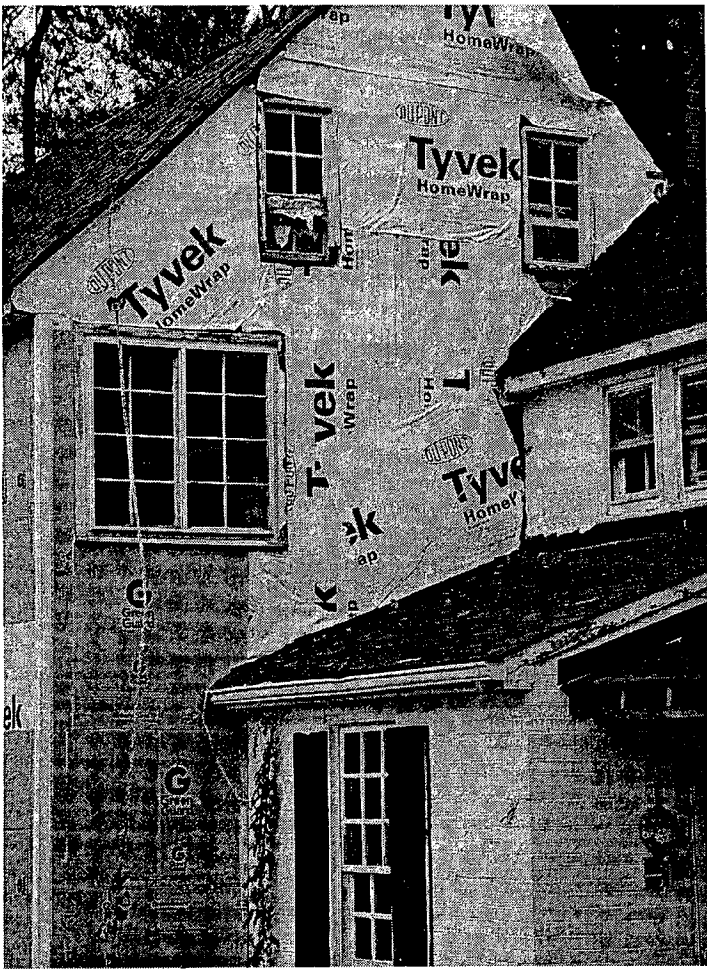
Detail, Building A October 24, 2003 North elevation
