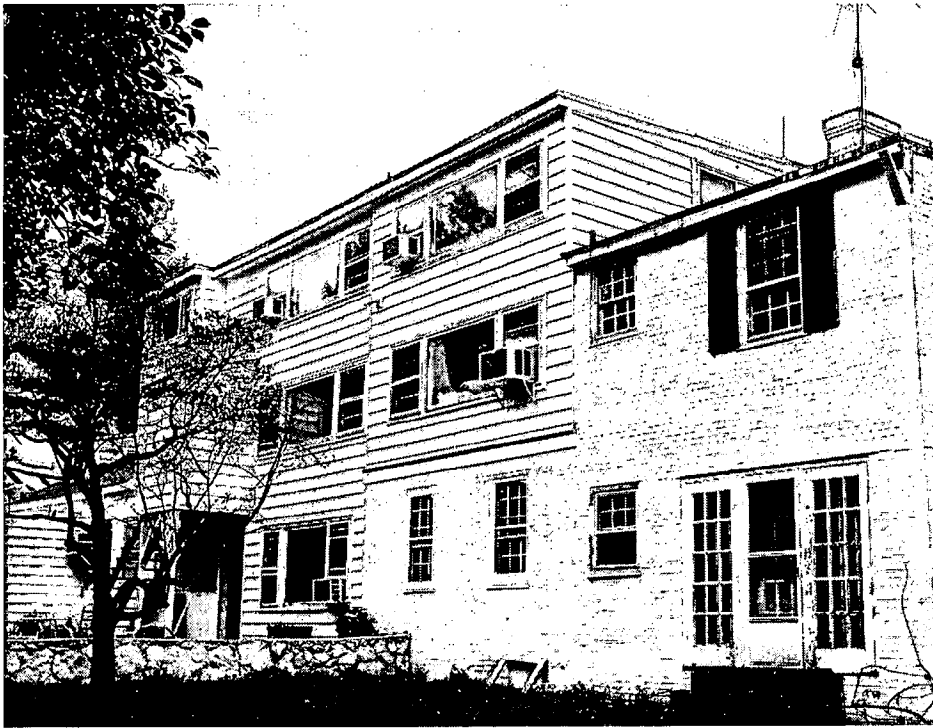
Building A West Elevation October 24, 2003 Showing 2-part construction of main house, brick addition at south end, raising of roof to include rear, 3rd story, and installation of multiple picture windows. October 24, 2003
