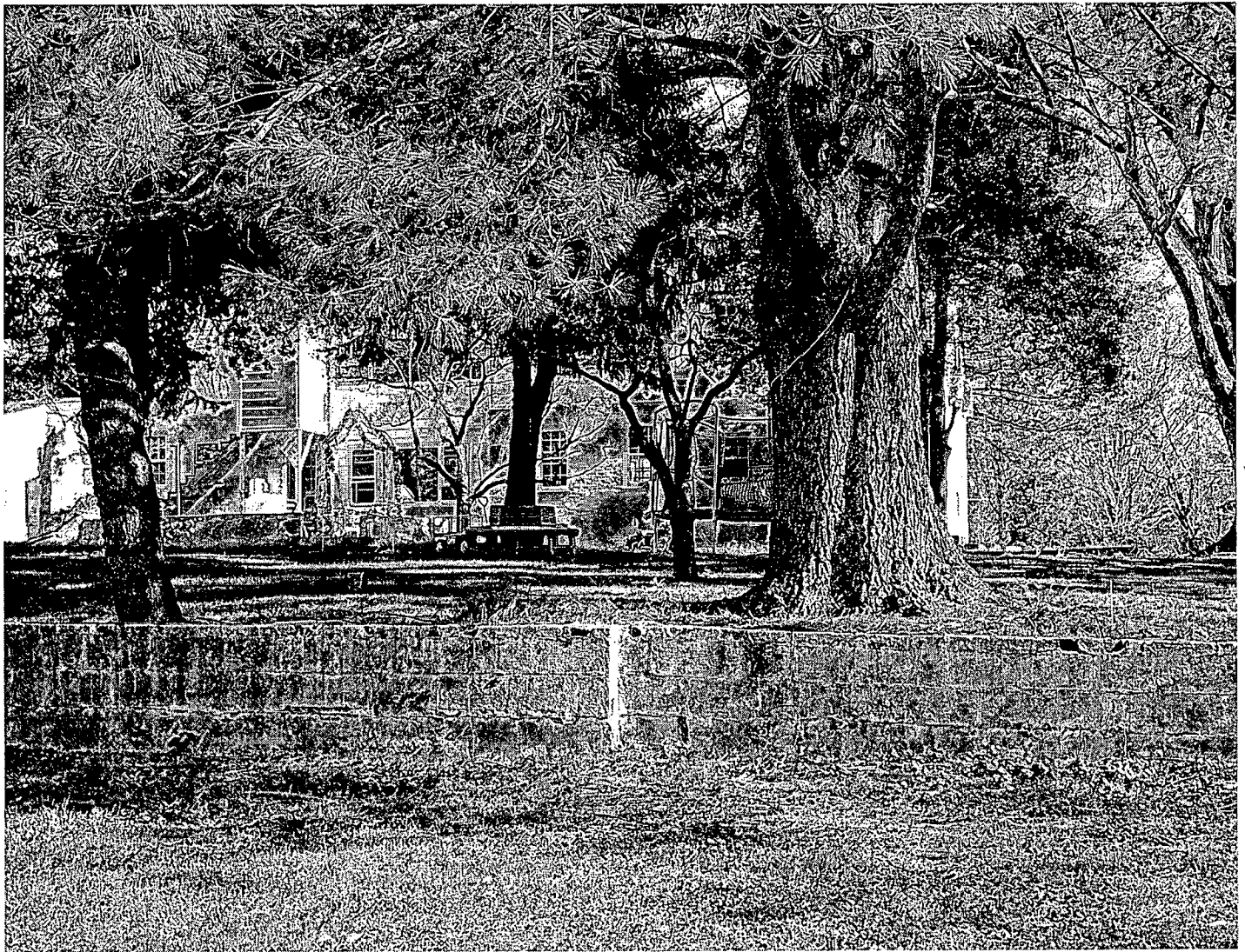
Ha-ha Wall now covered in Concrete block Nov. 2003
