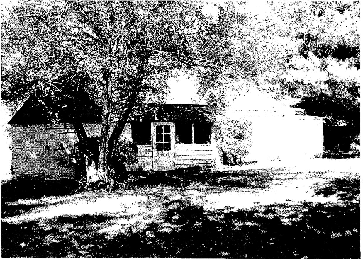
Building D Smokehouses Attached by Breezeway May 1990
