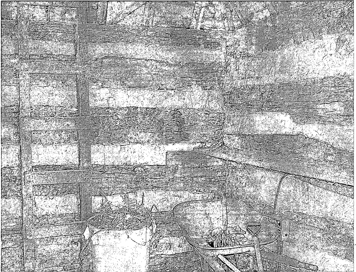
Building D Interior of Smokehouse Nov. 2003
