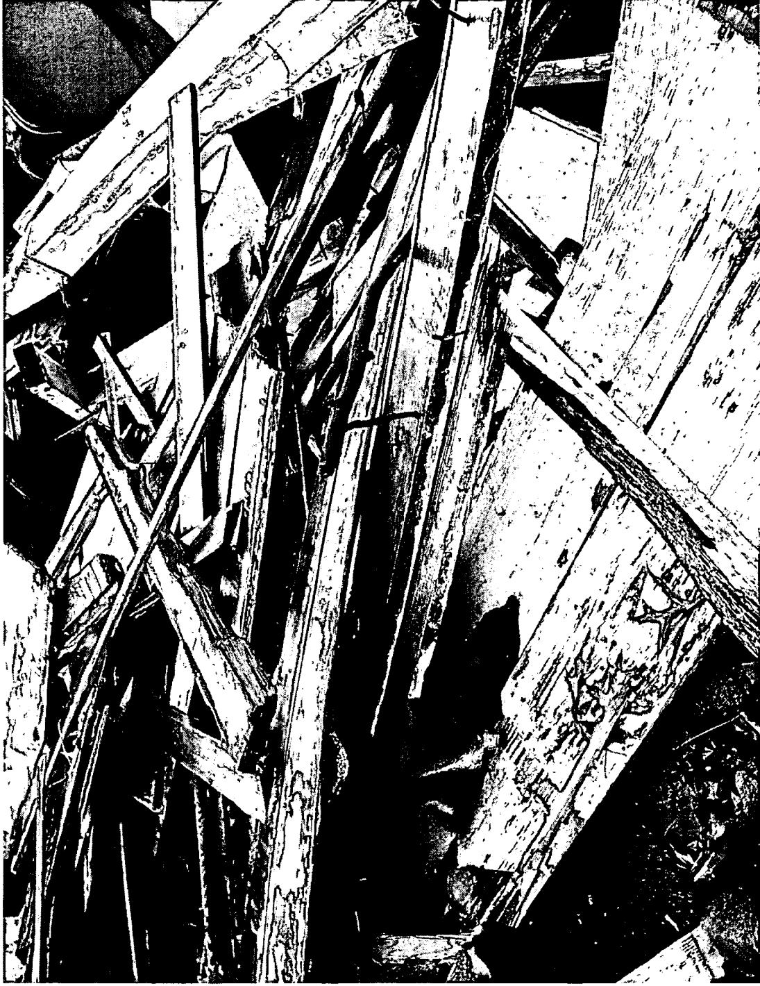
Building E Debris Pile Cleanup Showing fencing and clapboard Removed and stacked, October 24, 2003
