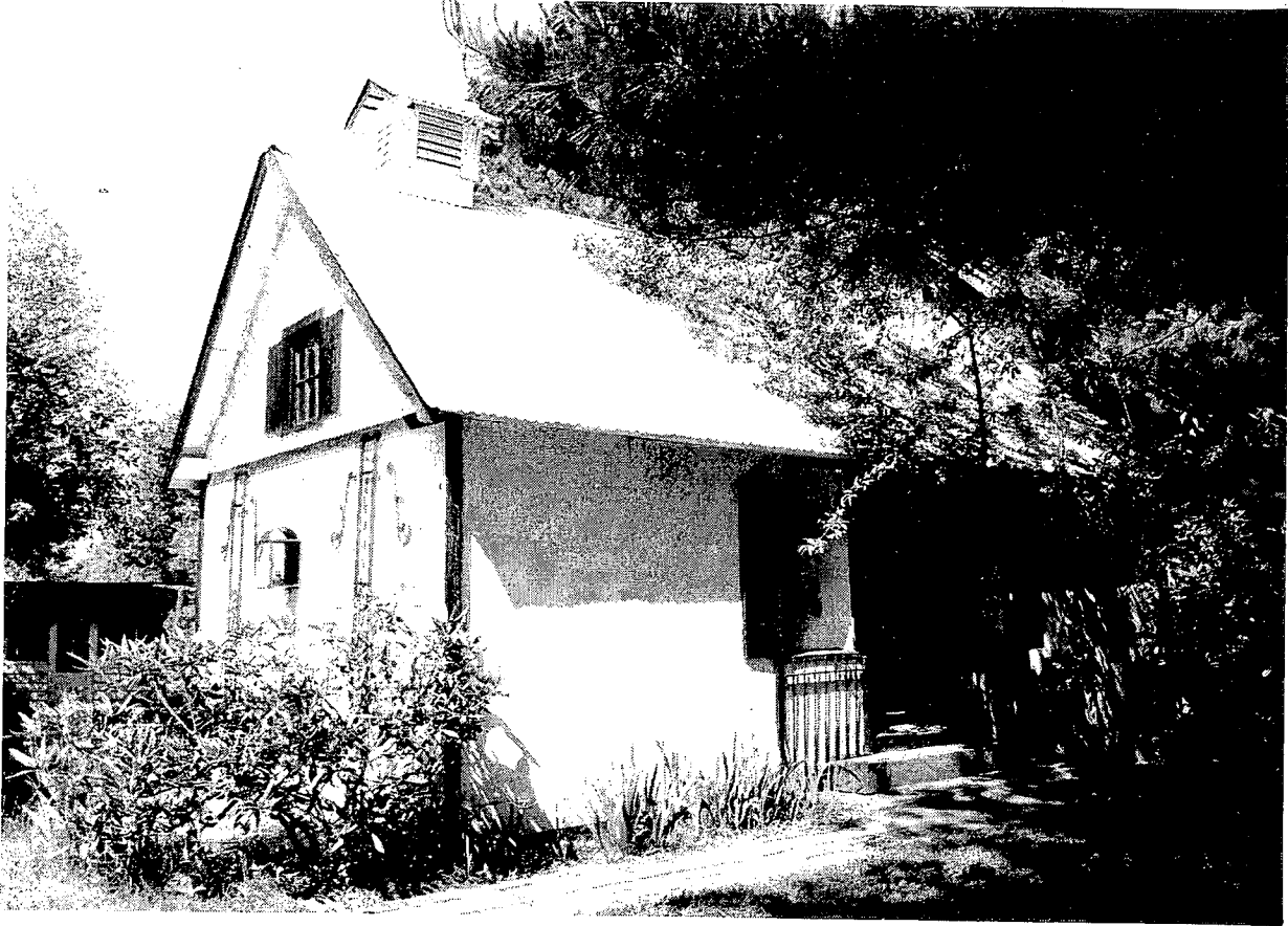
Building C Granary May 1990
