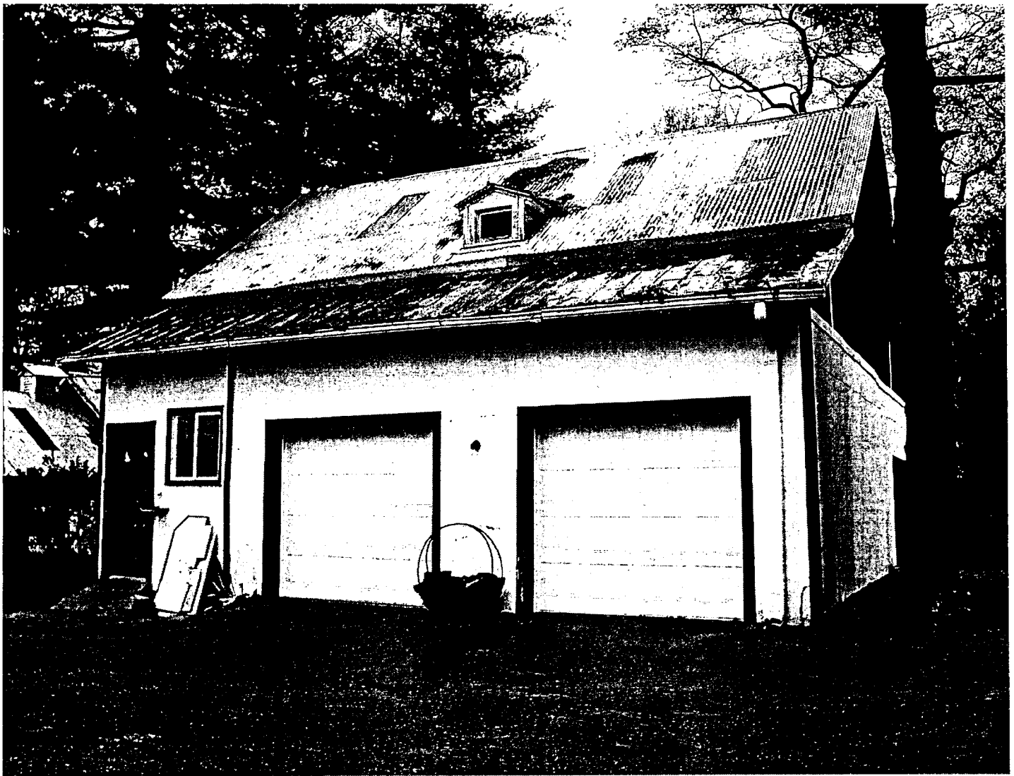
Building B Garage / Former Barn or Garage Structure covered in plywood / Homasote, (fiberboard) October 29, 2003
