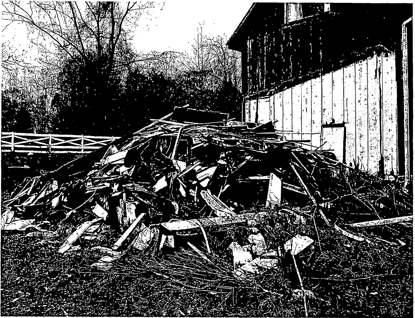
Building E Barn/Chicken Coop October 24, 2003 Showing collapse of attached stable and its ghost line and debris pile.
