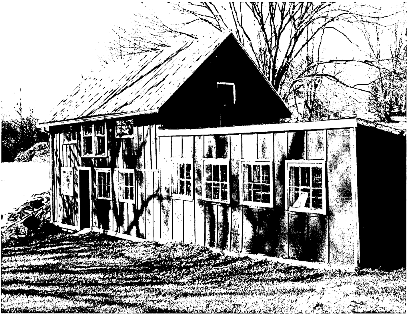
Building E Barn/Chicken Coop Nov. 2003
