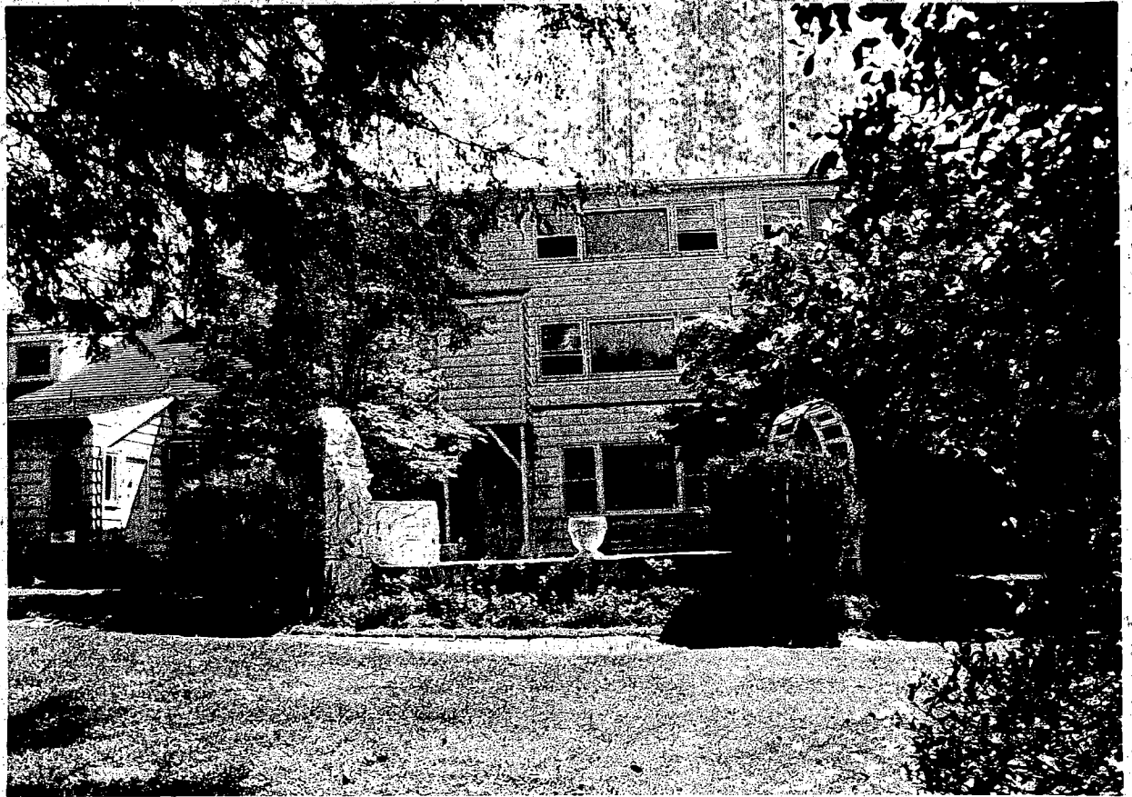
Building A Rear Elevation May 1990
