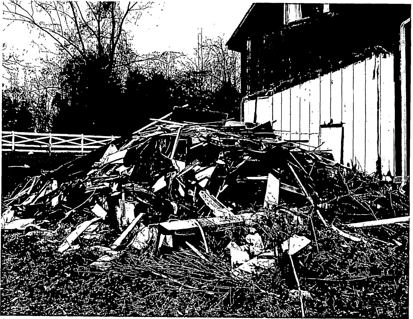
Building E Barn/Chicken Coop October 24, 2003 Showing collapse of attached stable and its ghost line and debris pile.
