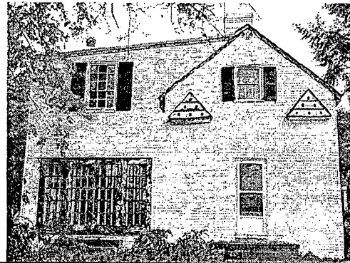
Brick Addition, South Side
