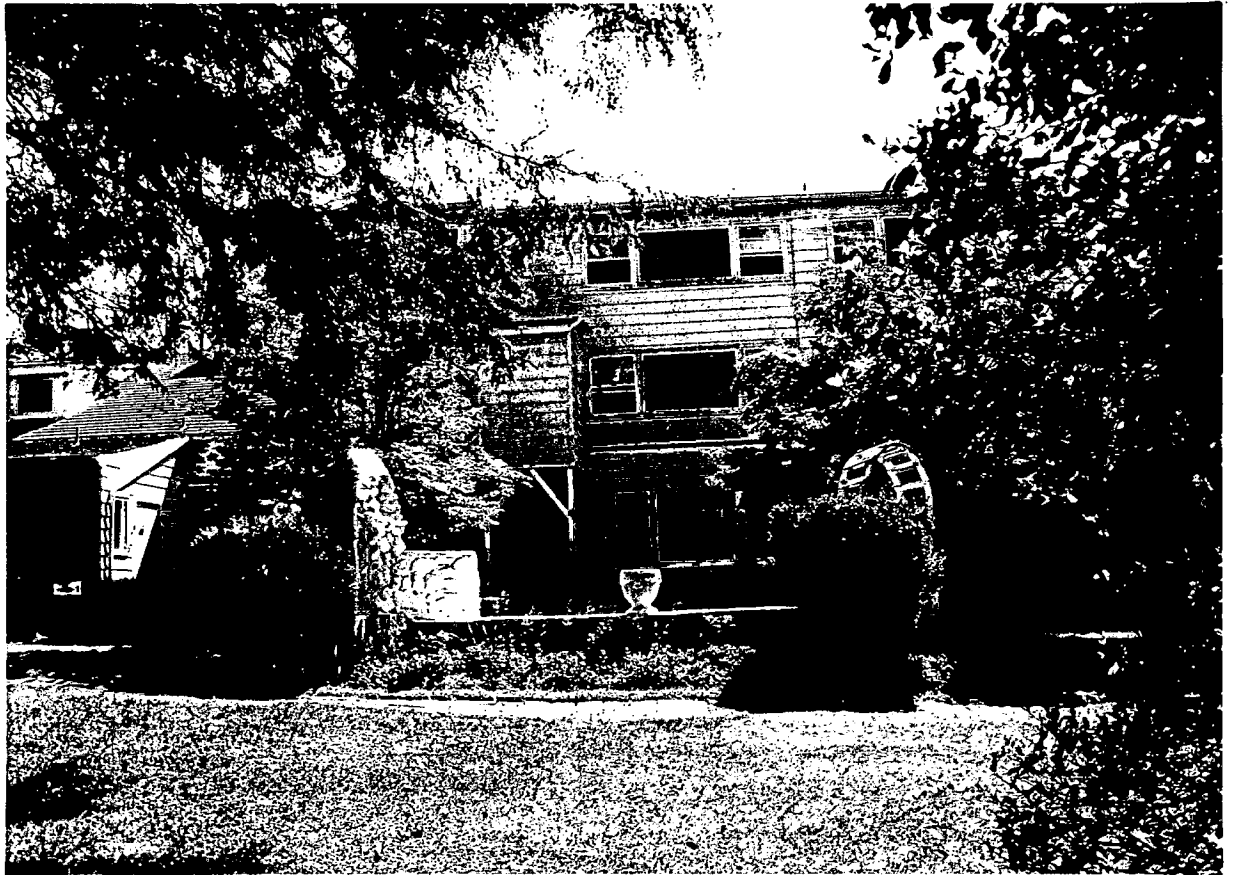
Building A Rear Elevation May 1990 (50)
