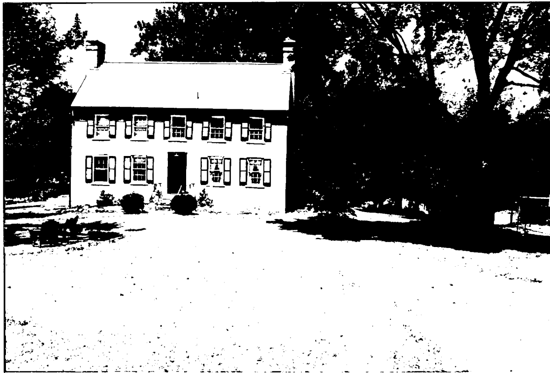
East side of loop driveway
