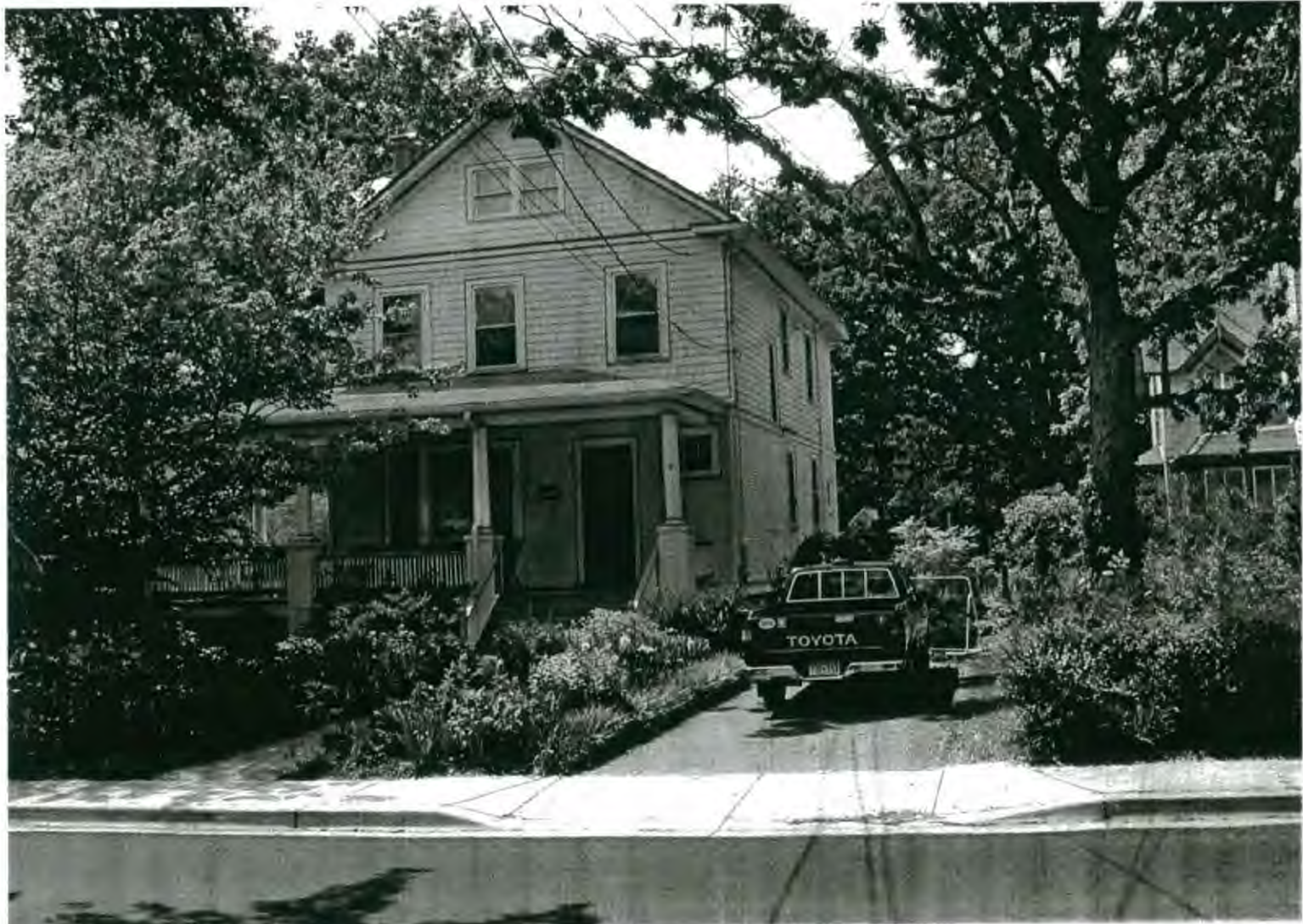
7112 Maple Avenue View of Property Adjacent to Halstead Residence
