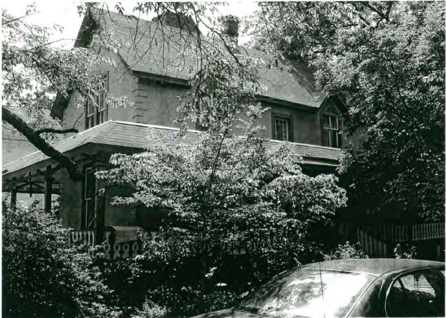
Halstead Residence 7116 Maple Avenue View of Right Side Facade
