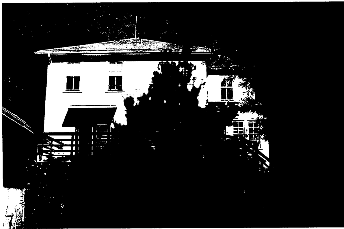
REAR ELEVATION (SOUTH-EAST)
