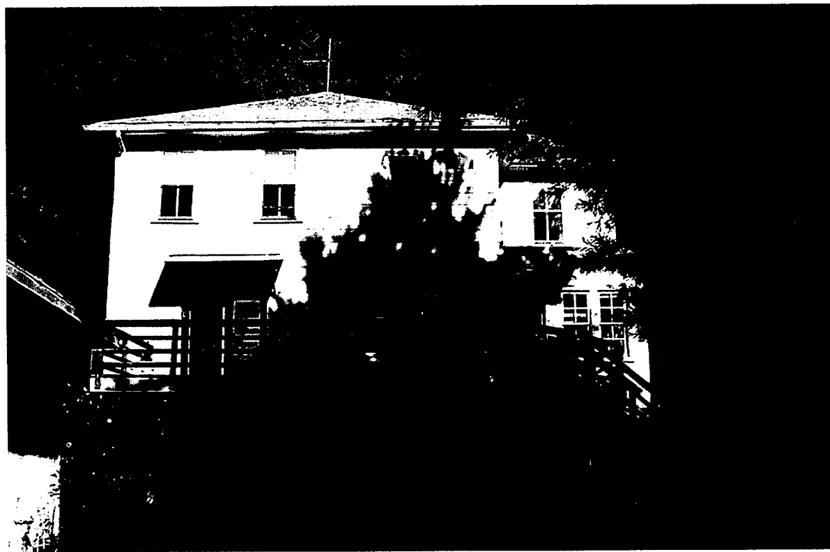
REAR ELEVATION (SOUTH-EAST)
