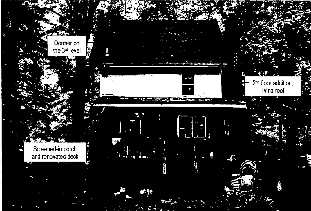
Fig. 2. 7400 Maple Avenue, Takoma Park, MD 20912 Rear View (west-facing side) with details of affected portions
