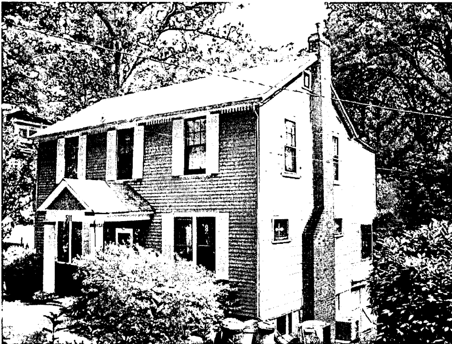
HERMAN RESIDENCE 511 NEW YORK AVE., TAKOMA PARK, MD 20912 VIEW FROM RIGHT OF WAY
