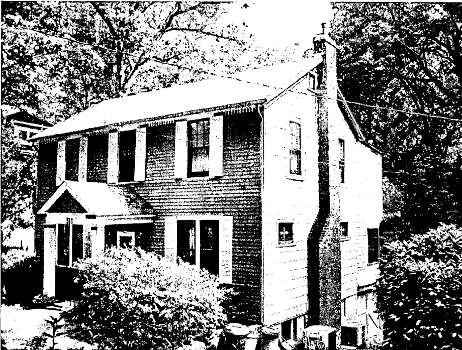
HERMAN RESIDENCE 511 NEW YORK AVE., TAKOMA PARK, MD 20912 VIEW FROM RIGHT OF WAY
