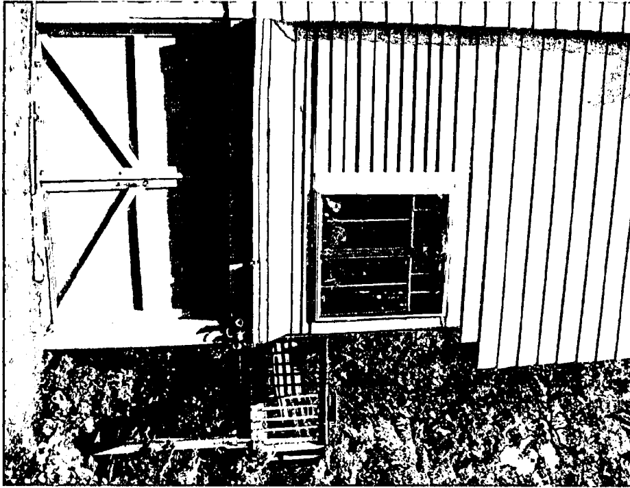
HERMAN RESIDENCE 511 NEW YORK AVE., TAKOMA PARK, MD 20912 REAR CORNER OF SIDE ELEVATION
