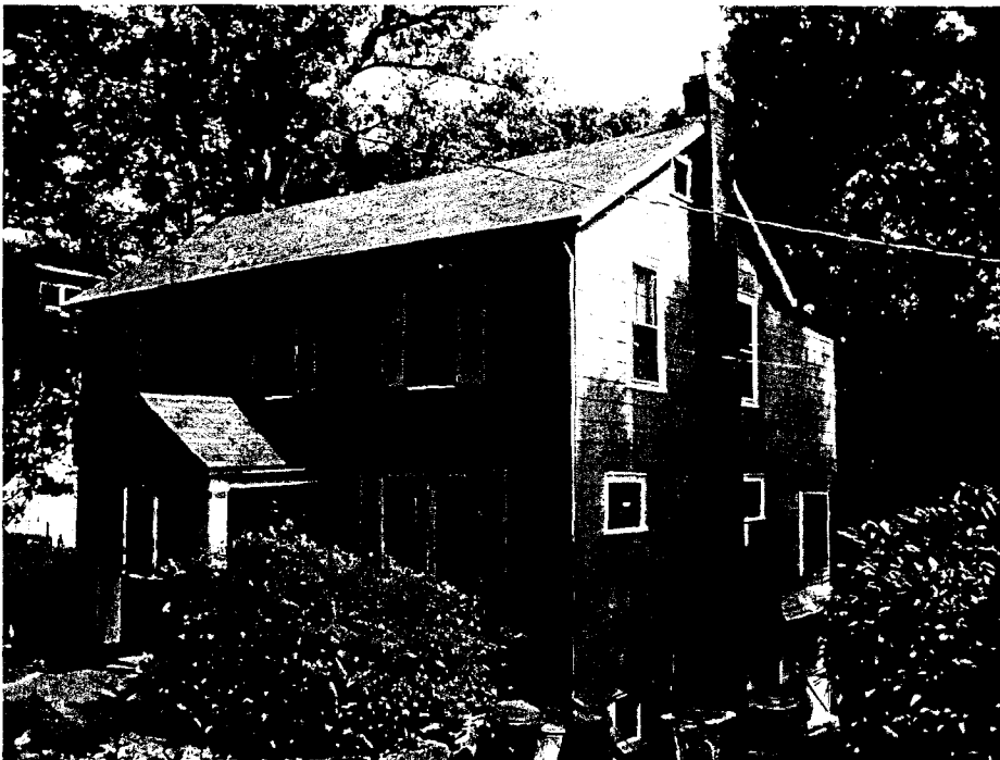
HERMAN RESIDENCE 511 NEW YORK AVE., TAKOMA PARK, MD 20912 VIEW FROM RIGHT OF WAY
