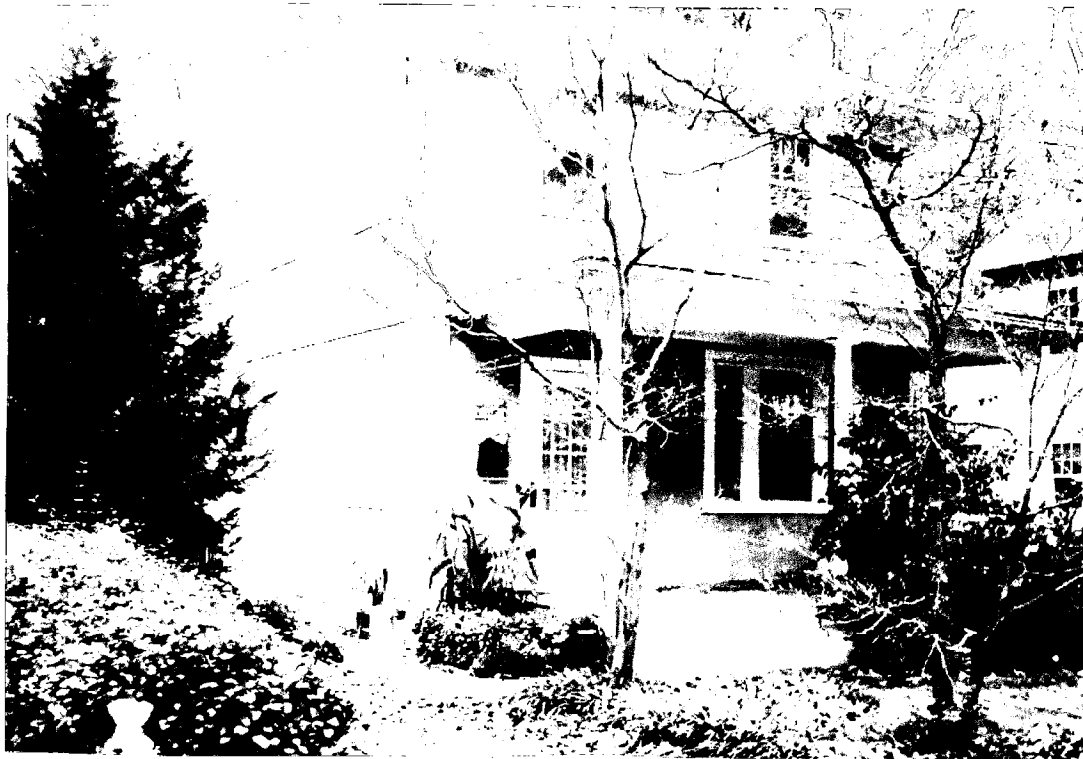
Detail: View of 7304 Maple Ave. (note siding over stucco)
