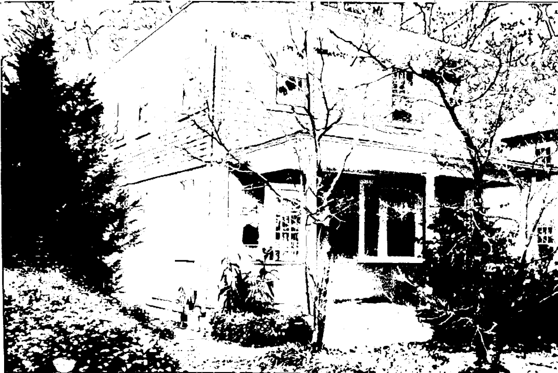
Detail: View of 7304 Maple Ave. (note siding over stucco)
