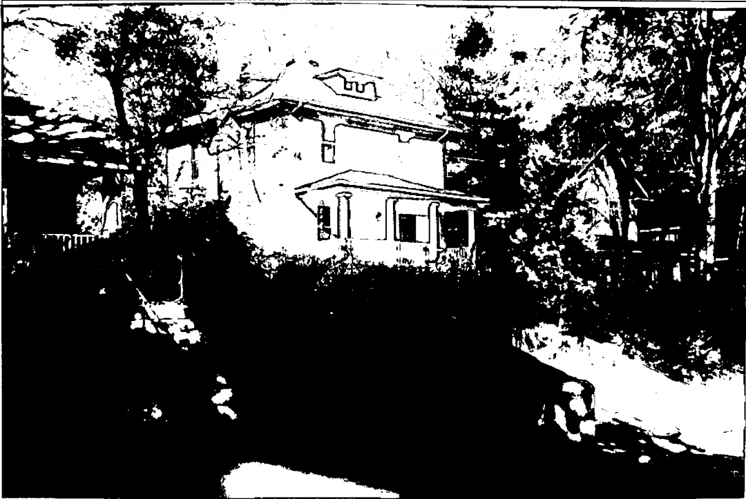
Detail: View from South-east
