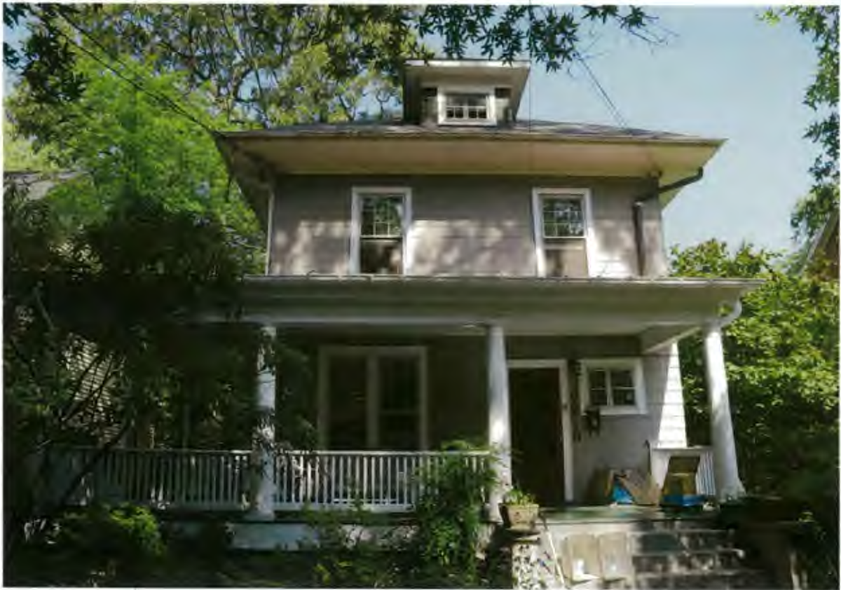
view of southeast face from street (to remain)
