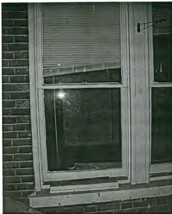
Front Window view 1
