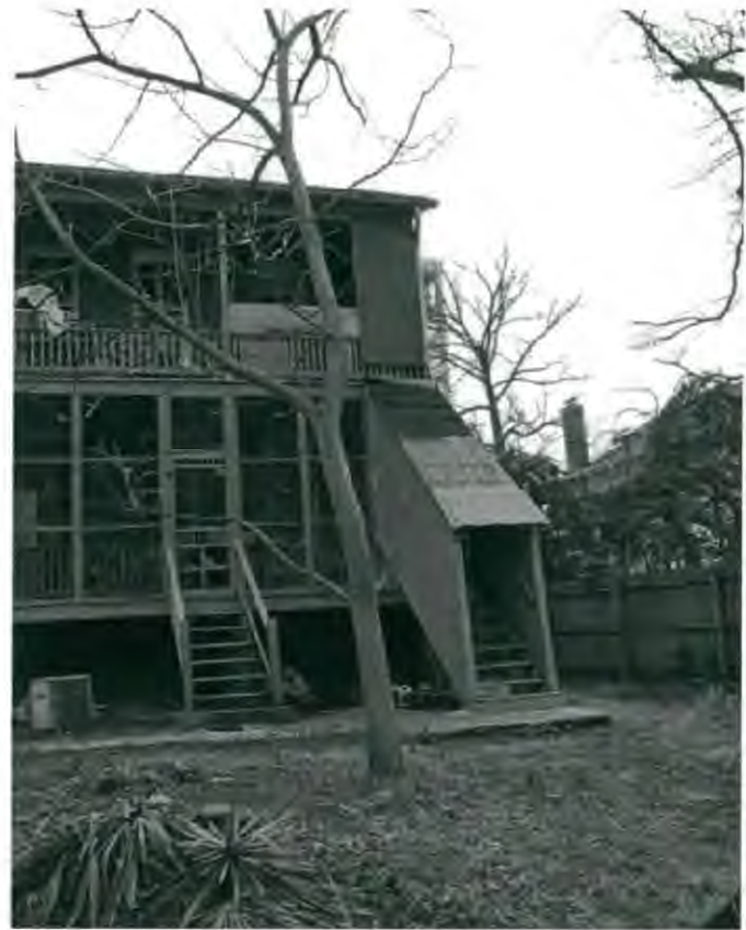
7102 stairways to upper level
