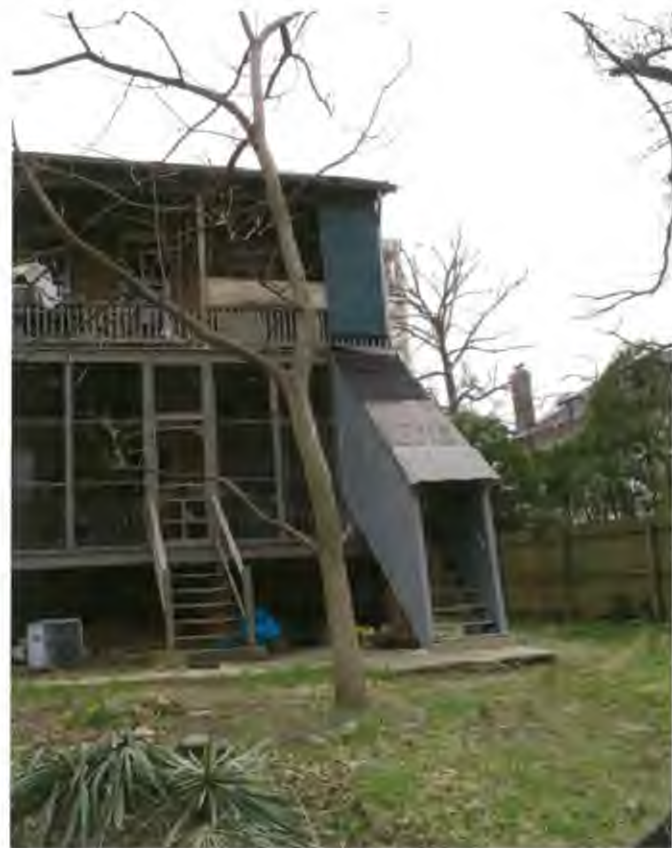
7102 stairways to upper level
