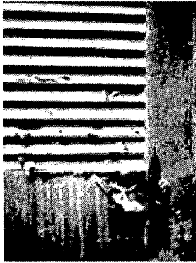
Here, a latex top coat was applied directly over old oil paint, resulting in intercoat peeling. The latex was unable to adhere. If latex is used over oil, an oil-base primer should be applied first. Photo: Mary L. Oehrlein, AIA.
