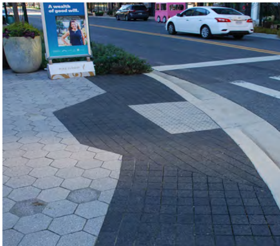
Figure 15: Paving at Pike & Rose clearly demarcates transitions between the street and frontage zone.
