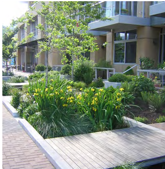
Figure 76: Examples of bioretention and stormwater management planters.
