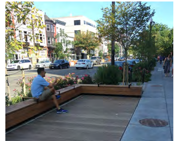
Figure 43: Example of a curb extension near an intersection to accommodate a parklet for outdoor seating.
