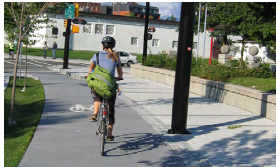
Example of a raised and separated bike lane with planting buffer, as recommended along Spring Street extension
